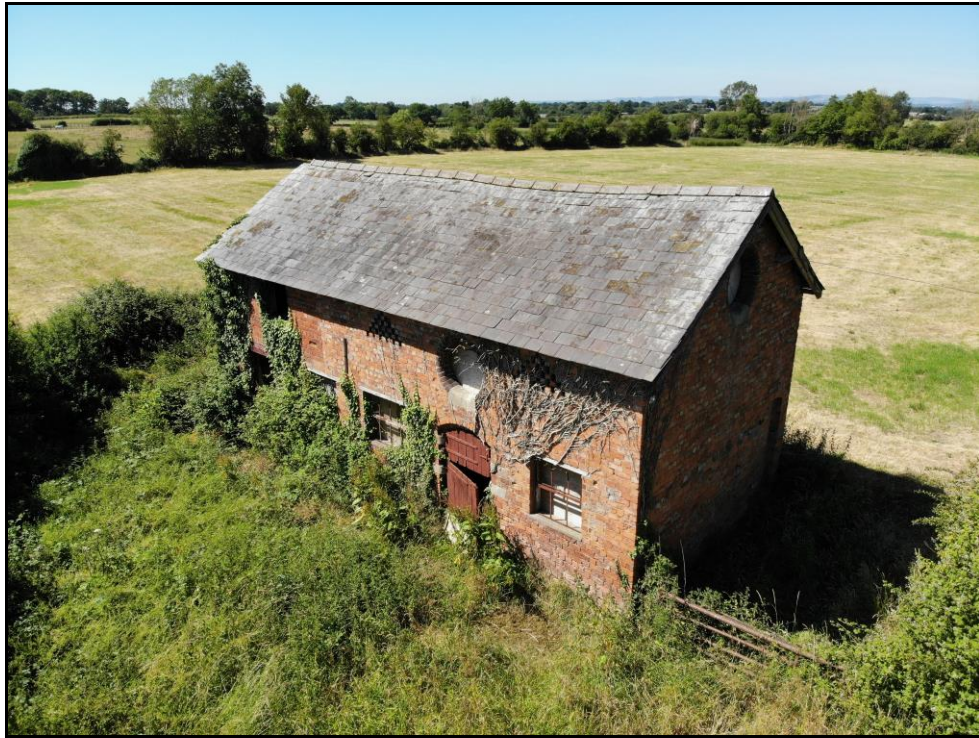
Photograph 9 showing the barn
