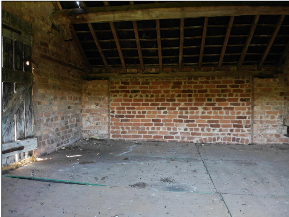
Photograph 12 showing the first floor of the barn
