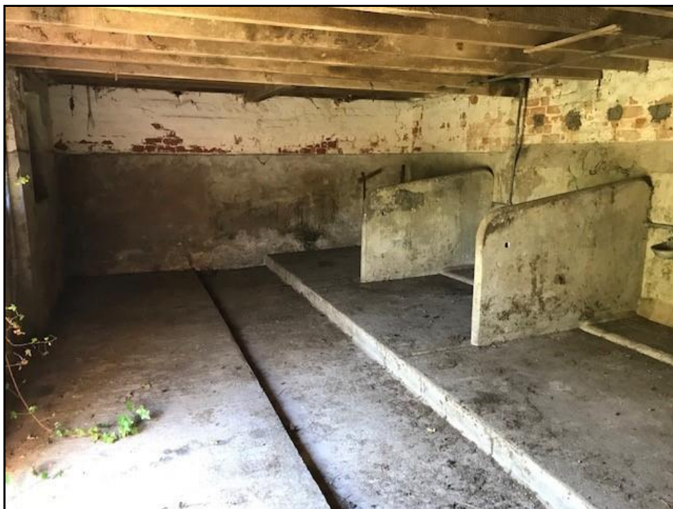
Photograph 11 showing the ground floor of the barn
