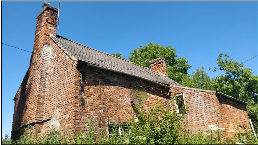
Photograph 2 showing the rear of the detached dwelling
