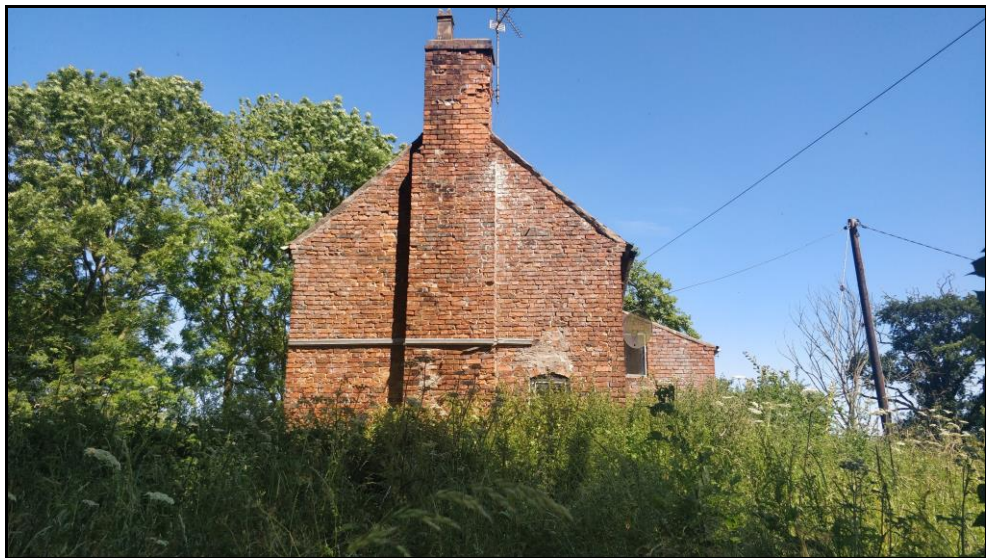
Photograph 3 showing the gable end and chimney stack
