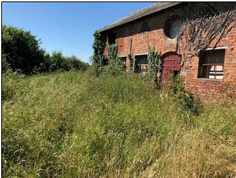
Photograph 10 showing the front of the barn
