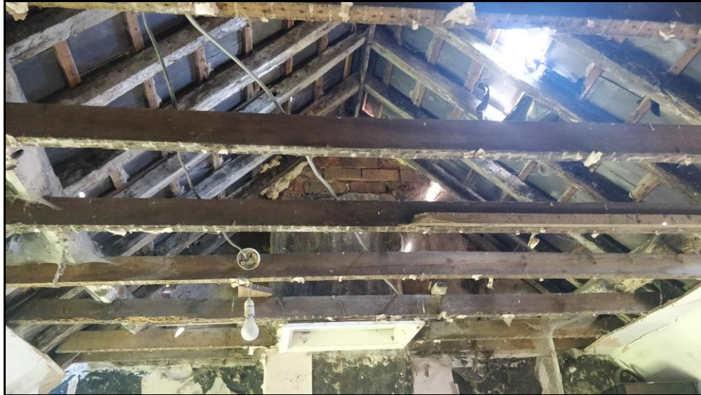
Photograph 6 showing the roof and ceiling joists
