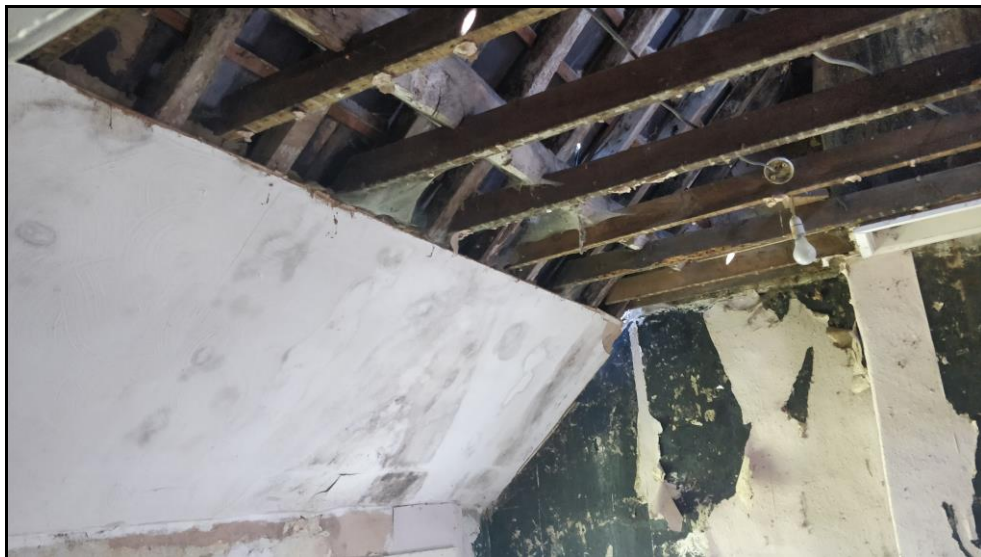
Photograph 7 showing plasterboard and wooden beams
