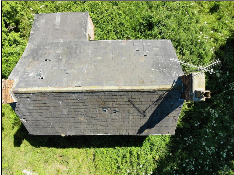
Photograph 4 showing the roof of the farmhouse
