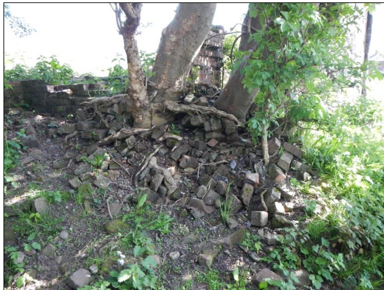
Figure 10: Rubble pile adjacent to brick structure (TN01)
