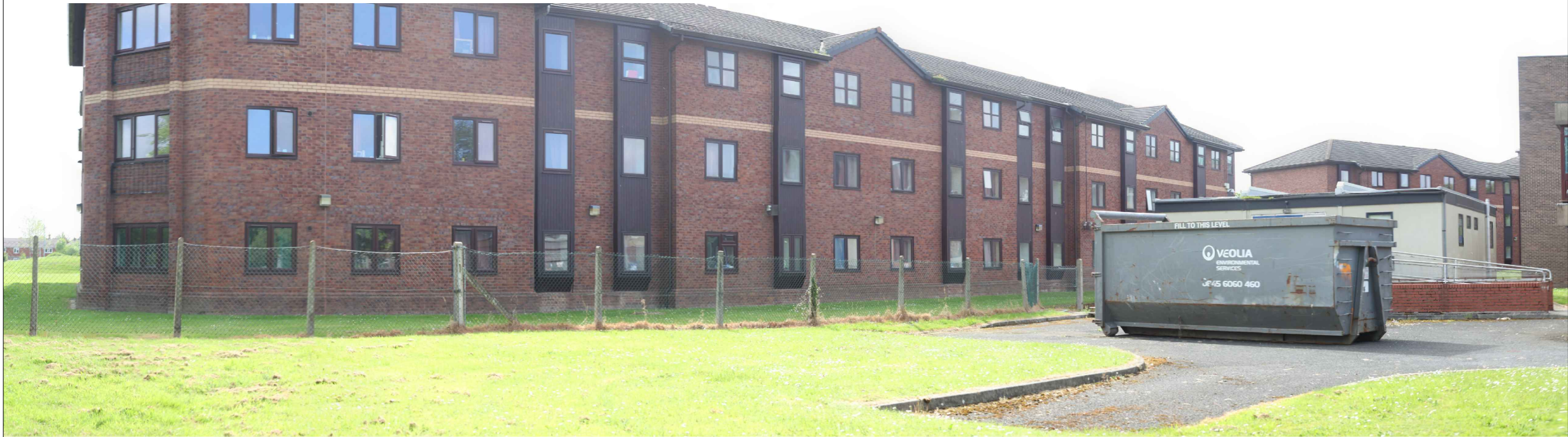
Photograph 2: View looking south-west into the Site from the entrance to the Tennis Centre
