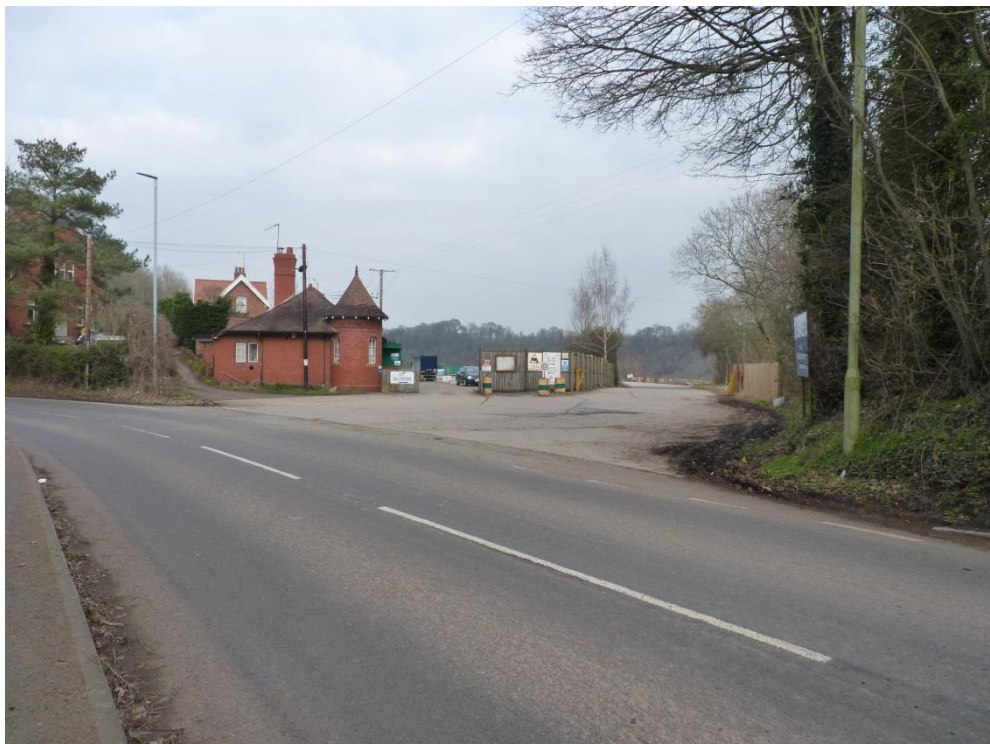
PLATE 3: THE FORMER PEN Y BONT BRICK AND TILE COMPANY OFFICE AND SITE ENTRANCE
