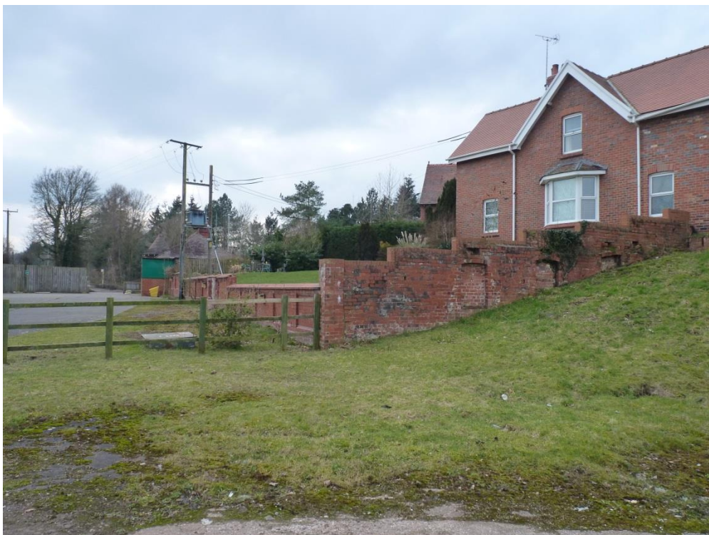
PLATE 5: FRAGMENTARY REMAINS OF BRICKWORK
