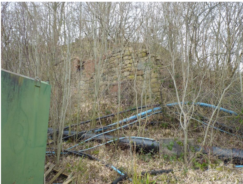
PLATE 7: MASONRY IN EARTH BANK
