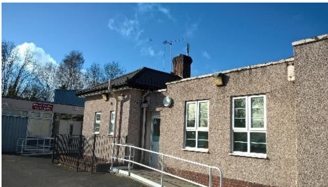
PICTURES 5 AND 6. THE DODD'S LANE STUDENT CENTRE BUILDING. NOTE RENDERED BRICK AND PREFABRICATED METAL CONSTRUCTION.
