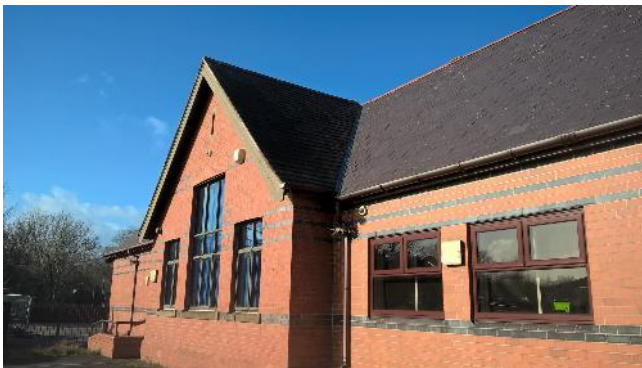
PICTURE 1. SOUTH ELEVATION OF BUILDING 1 (WHERE EXTENSION WILL TIE IN).
