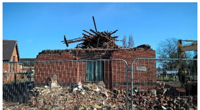
PICTURE 18. THE PARTLY DEMOLISHED BUILDING 2.
