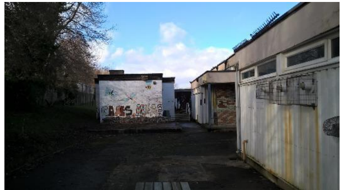
PICTURES 21 AND 22. BUILDING 4, PREFABRICATED CORRUGATED SHEETS AND WOOD TO THE SOUTH.
