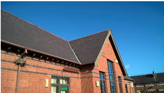
PICTURE 7. SOUTH ELEVATION OF BUILDING 1.
