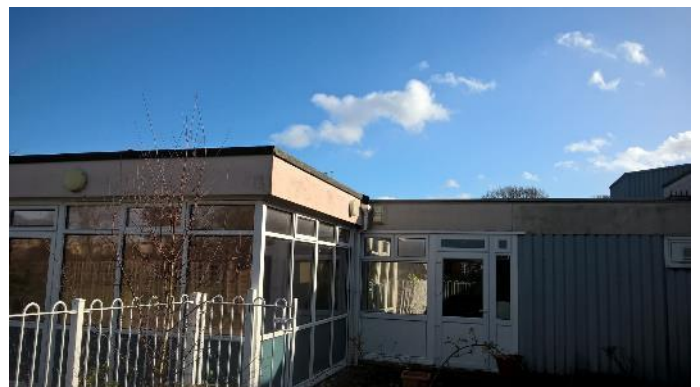
PICTURE 24. FLAT ROOFED SECTION OF BUILDING 4.
