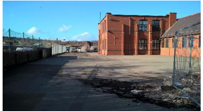
PICTURE 28. HARDSTANDING AROUND BUILDING 1
