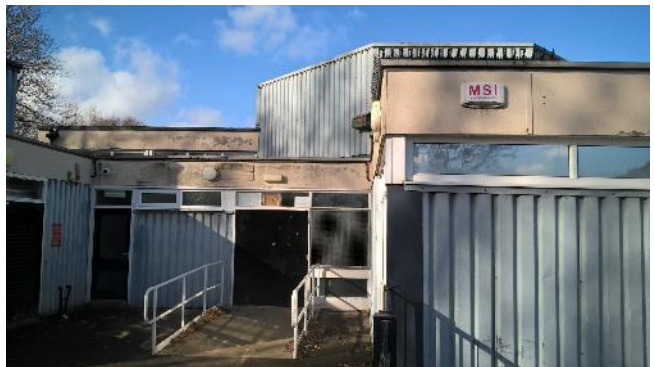
PICTURES 5 AND 6. THE DODD'S LANE STUDENT CENTRE BUILDING. NOTE RENDERED BRICK AND PREFABRICATED METAL CONSTRUCTION.
