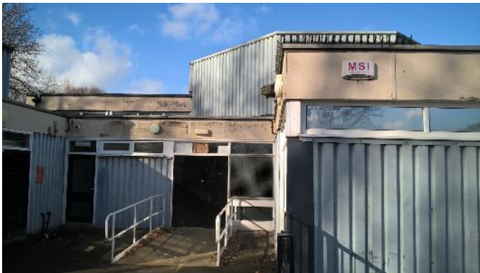
PICTURES 21 AND 22. BUILDING 4, PREFABRICATED CORRUGATED SHEETS AND WOOD TO THE SOUTH.
