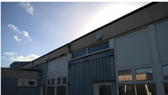
PICTURE 23. FLAT ROOFED SECTION OF BUILDING 4.
