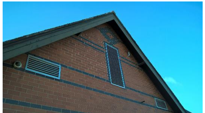
PICTURE 8. VENTS ON THE SOUTHWEST GABLE, BUILDING 1.
