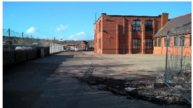
PICTURE 2. NORTHWEST SIDE OF BUILDING 1, INCLUDING TALL TWO STOREY EXTENSION.
