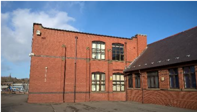
PICTURE 11. THE WESTERN TWO STOREY EXTENSION.
