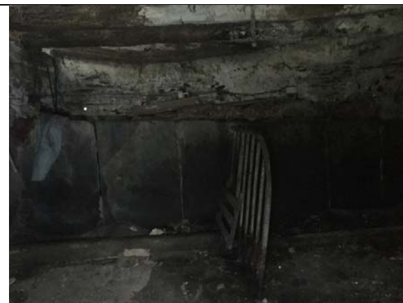
Plate 15: Holes in back wall
