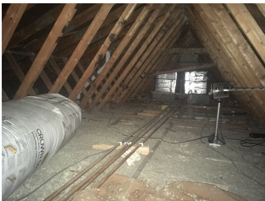
Plate 6: Roof void of building
