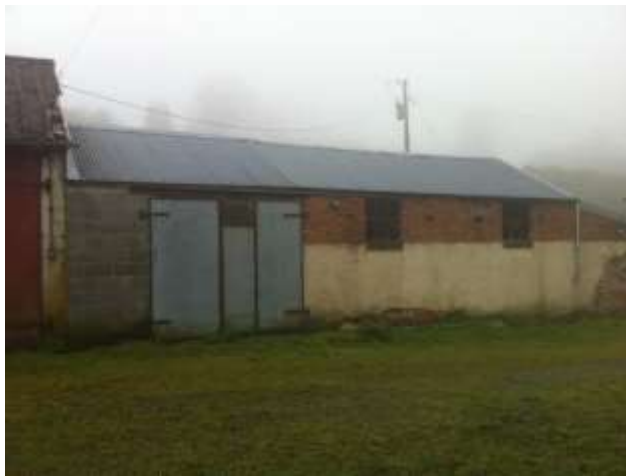
Photo B – Redundant Farm Building
