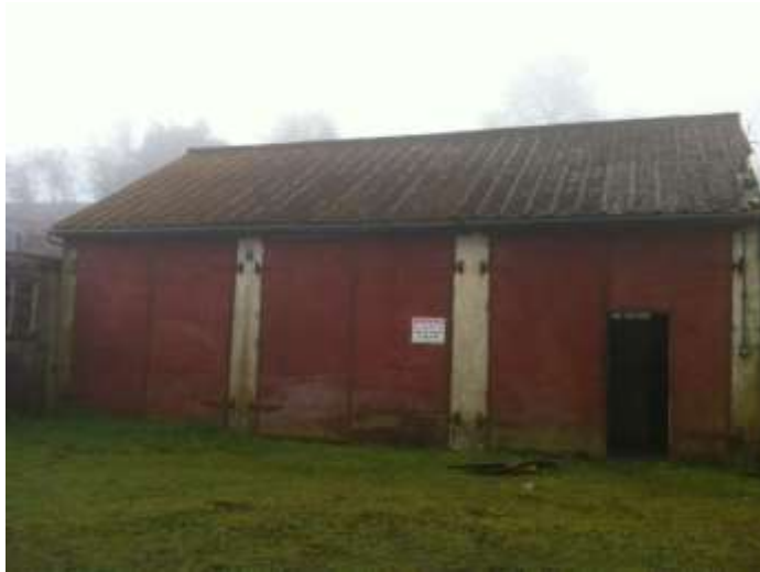
Photo A – Redundant Farm Building
