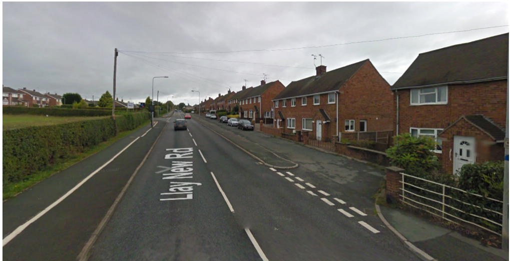
Figure 2: view northbound on Llay New Road (service road on right)
