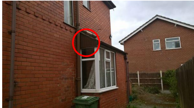
Plate 4.14: B2 – North-Western Extension With Barge Boards
