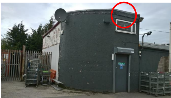
Plate 4.5: B1 – South-Western Elevation, Southern Corner, Showing Barge Board
