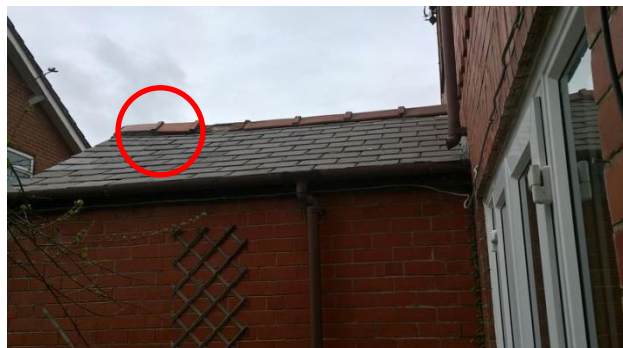
Plate 4.16: B2 – North-Western Extension With Barge Boards
