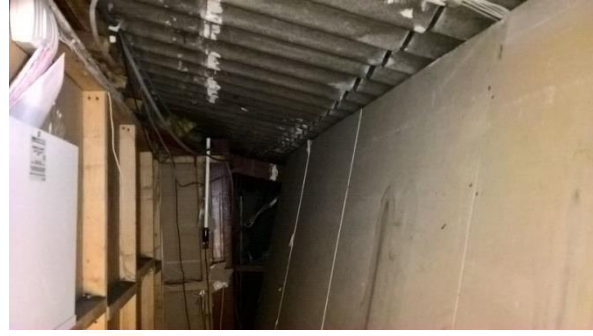
Plate 4.8: B1 – Further View of Roof Space
