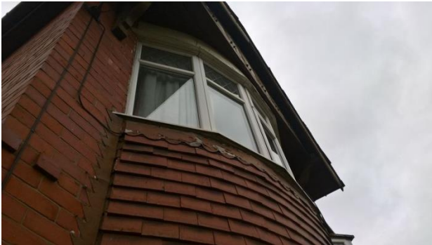
Plate 4.13: B2 – Hanging Tiles Between Bay Windows
