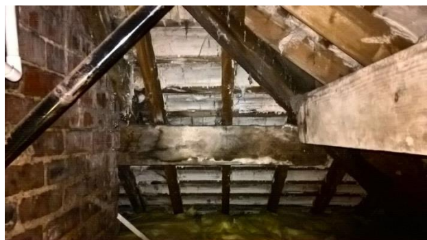
Plate 4.20: B2 – Brickwork of Chimney Stack
