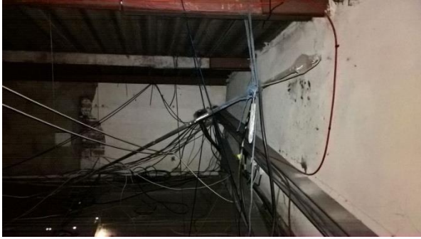
Plate 4.7: B1 – Roof Space
