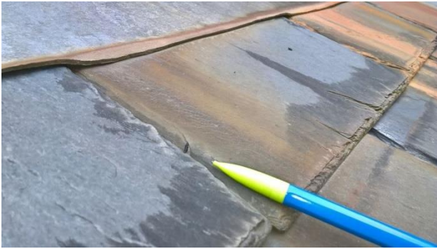
Plate 4.17: B2 – Bat Dropping on Coal Store
