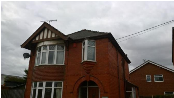
Plate 4.9: B2 – North-Eastern Elevation
