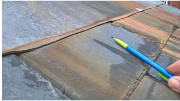
4.18: B2 – Second Bat Dropping on Coal Store
