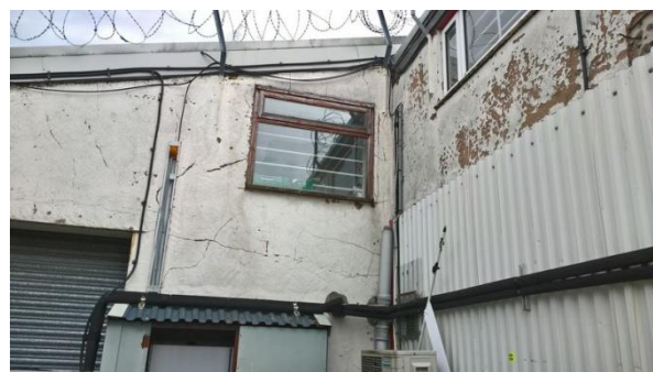
Plate 4.6: B1 – South-Western Elevation, Northern Corner
