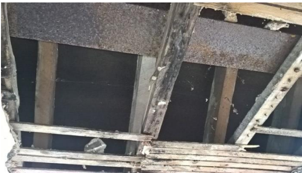
Plate 4.21: B2 – Internal Roof Space of Extension, Showing Felt Sarking
