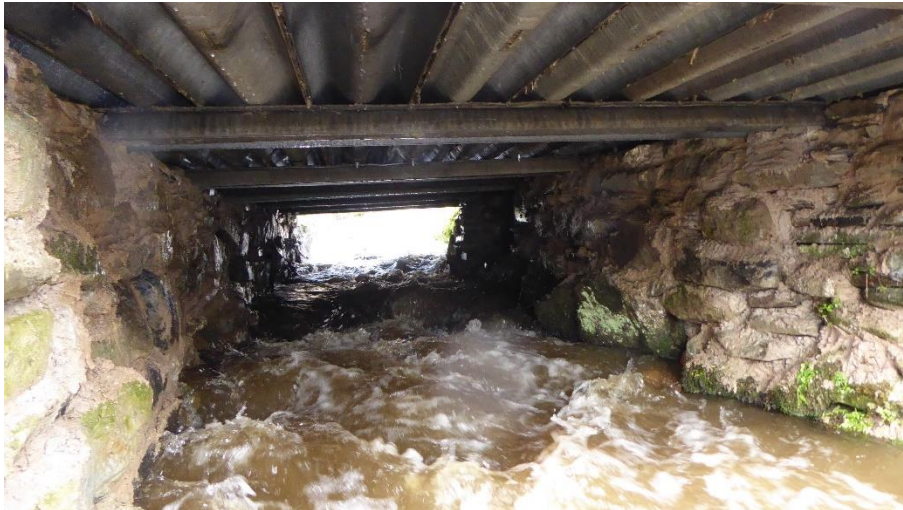
Figure 4.9. Underneath a bridge
