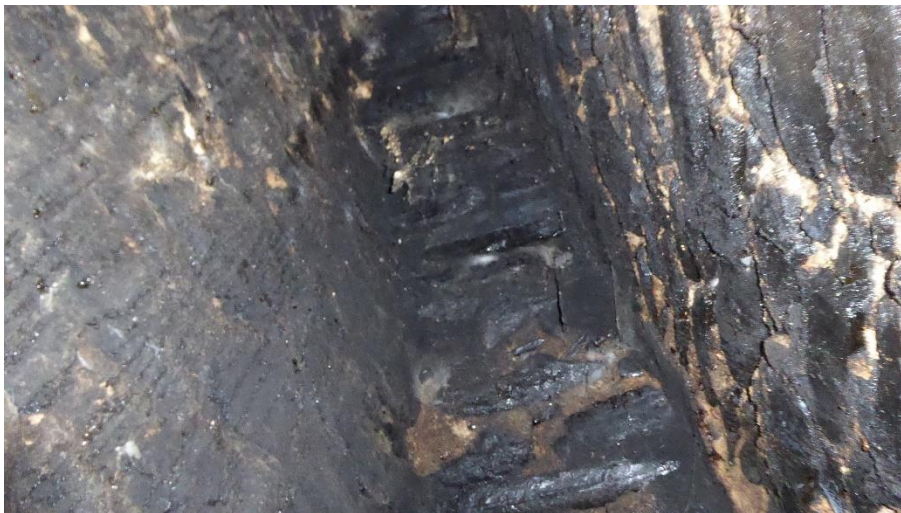
Figure 4.5. Inside the chimney
