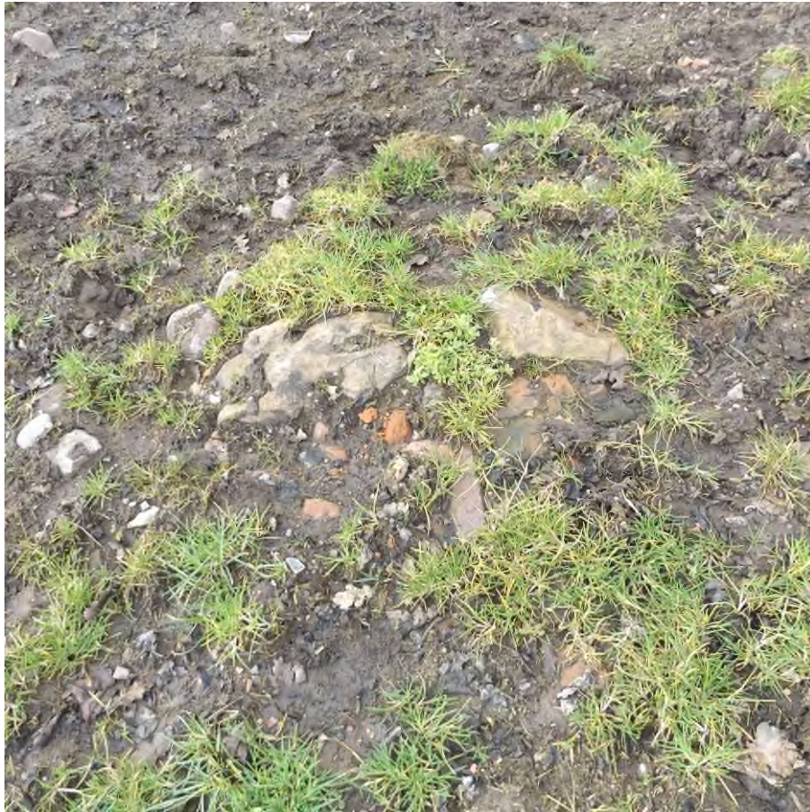
Above: There is already a layer of hard-core under the proposed car parking area.
