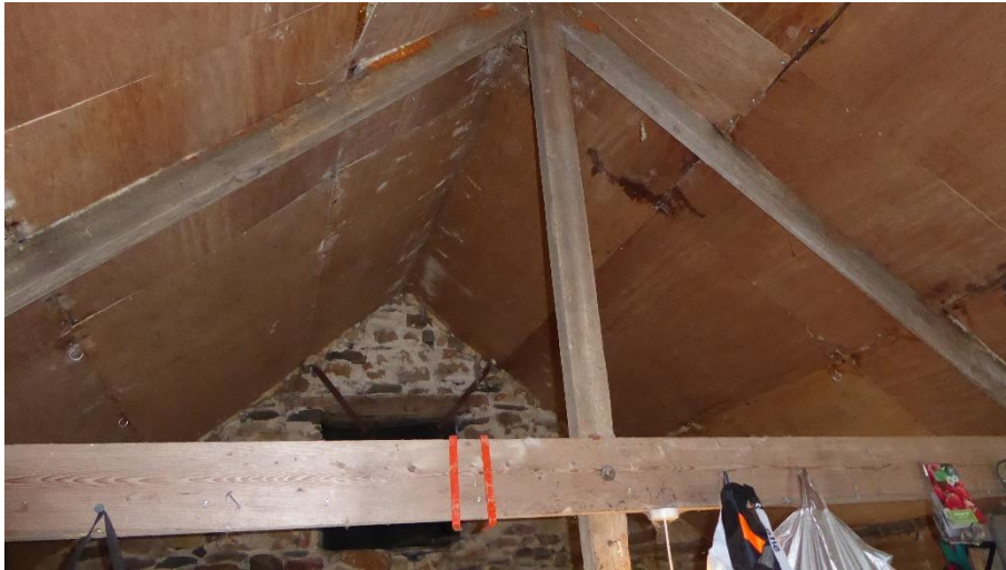
Figure 4.4. Wooden lining under northern roof
