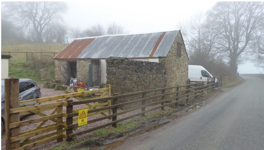
Figure 4.9. Wall seen extending from building
