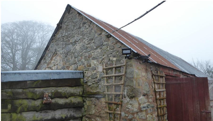
Figure 4.2. Southern gable end
