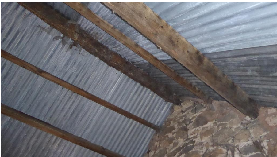
Figure 4.3. Roof over southern room
