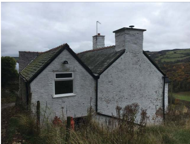
Photo 5: House viewed from the north.
