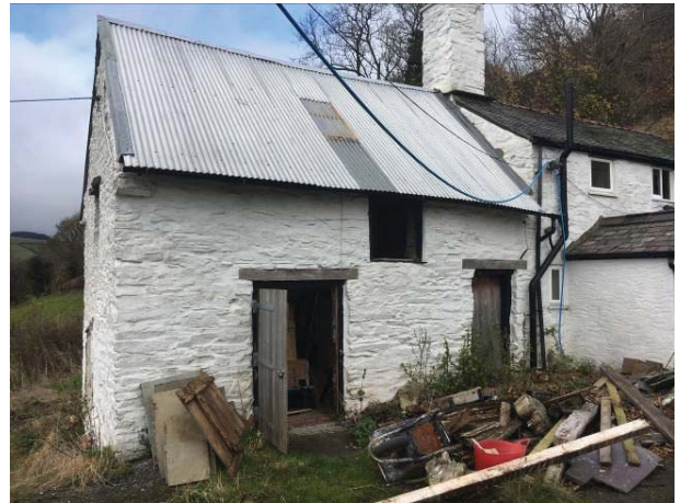
Photo 2: Hay barn viewed from the south east..
