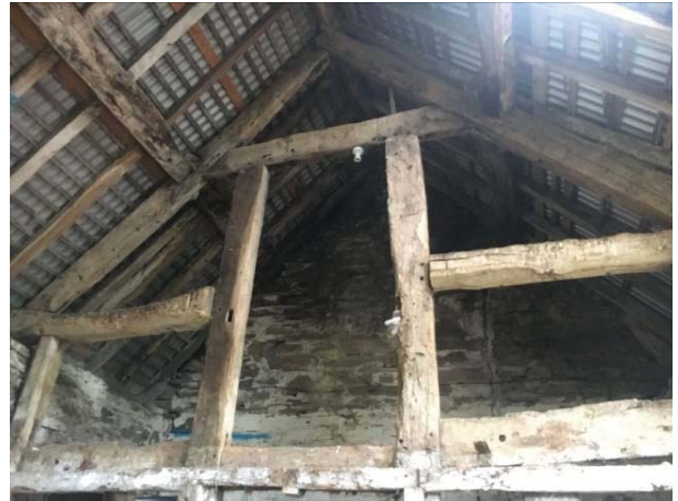
Photo 8: Internal view of hay barn.
