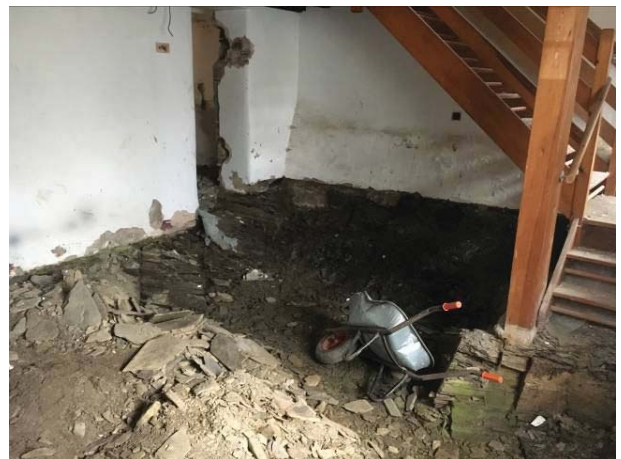
Photo 6: Internal view of house - ground floor.
