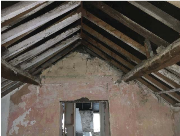
Photo 7: Internal view of house - upper room.
