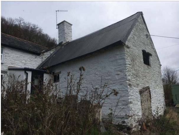
Photo 3: Hay Barn viewed from the west.
