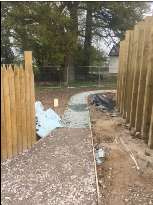
Photo 3 & 4 - Cellweb section within RPA of T24
