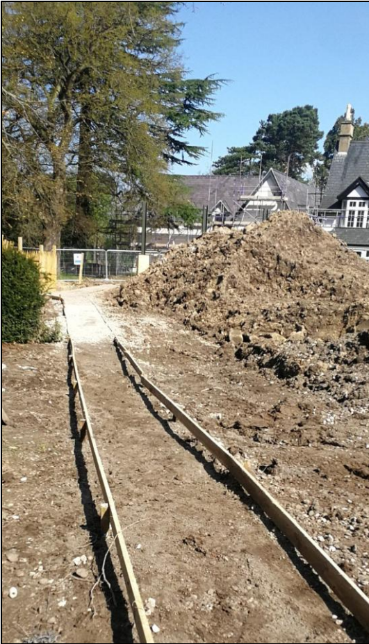
Photo 1 - No dig section prior to installation of Cellweb
