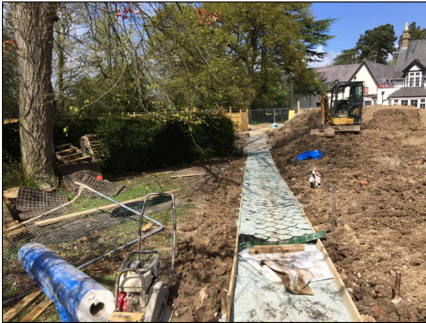
Photo 5 - Cellweb section within RPA of T25 & G1
