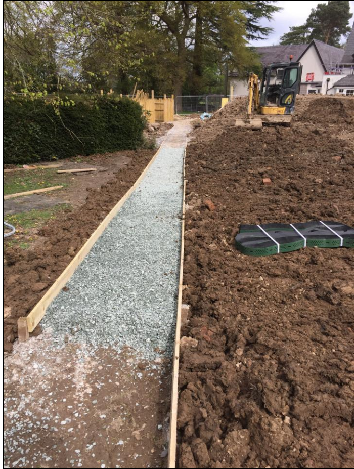
Photo 2 - Washed granite stone containing no-fines backfilled into cellweb
