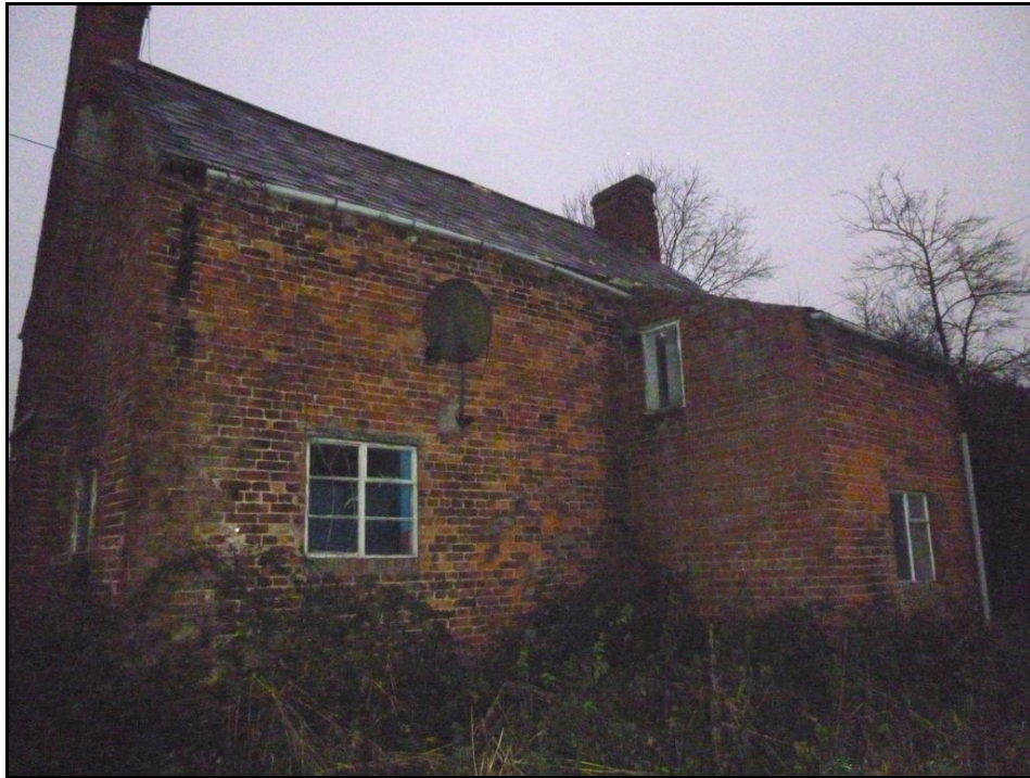
Photograph 2 showing the rear of the detached dwelling
