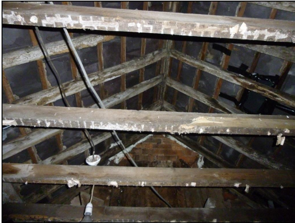
Photograph 3 showing the roof and ceiling joists
