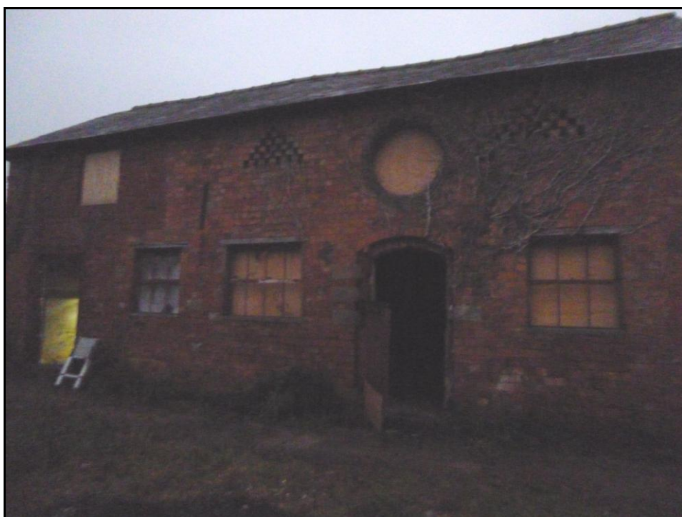
Photograph 8 showing the secured windows of the barn
