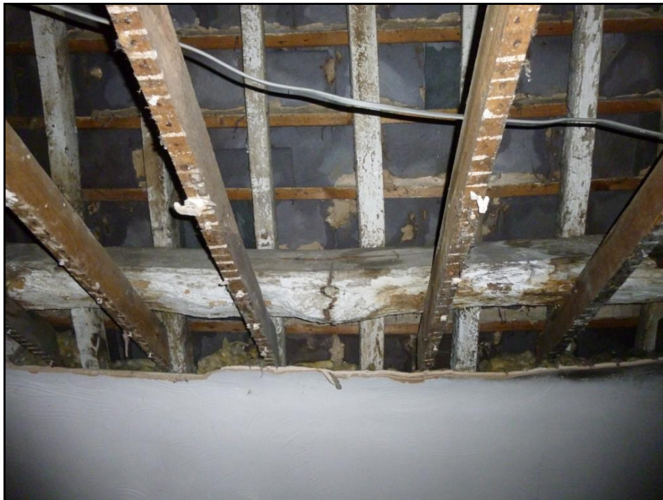
Photograph 4 showing roof tiles and wooden beams
