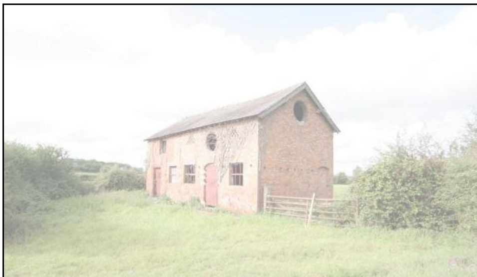
Photograph 7 showing the barn in the summer (taken from client stock)
