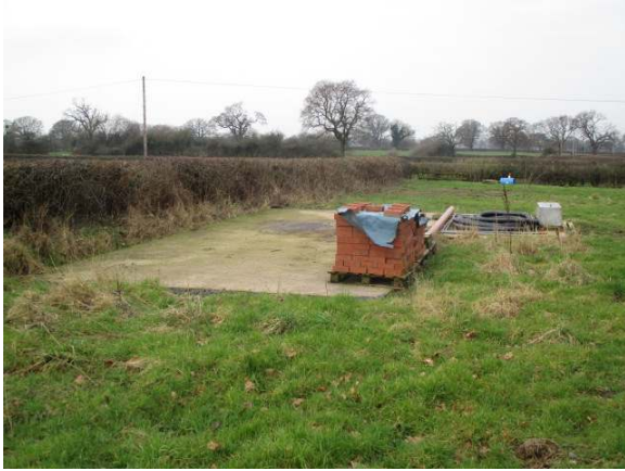
Plate 9. Area of hard standing for construction of timber stable building.
