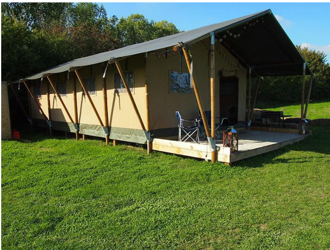
Fig. 3.2 Photograph example of safari tent
