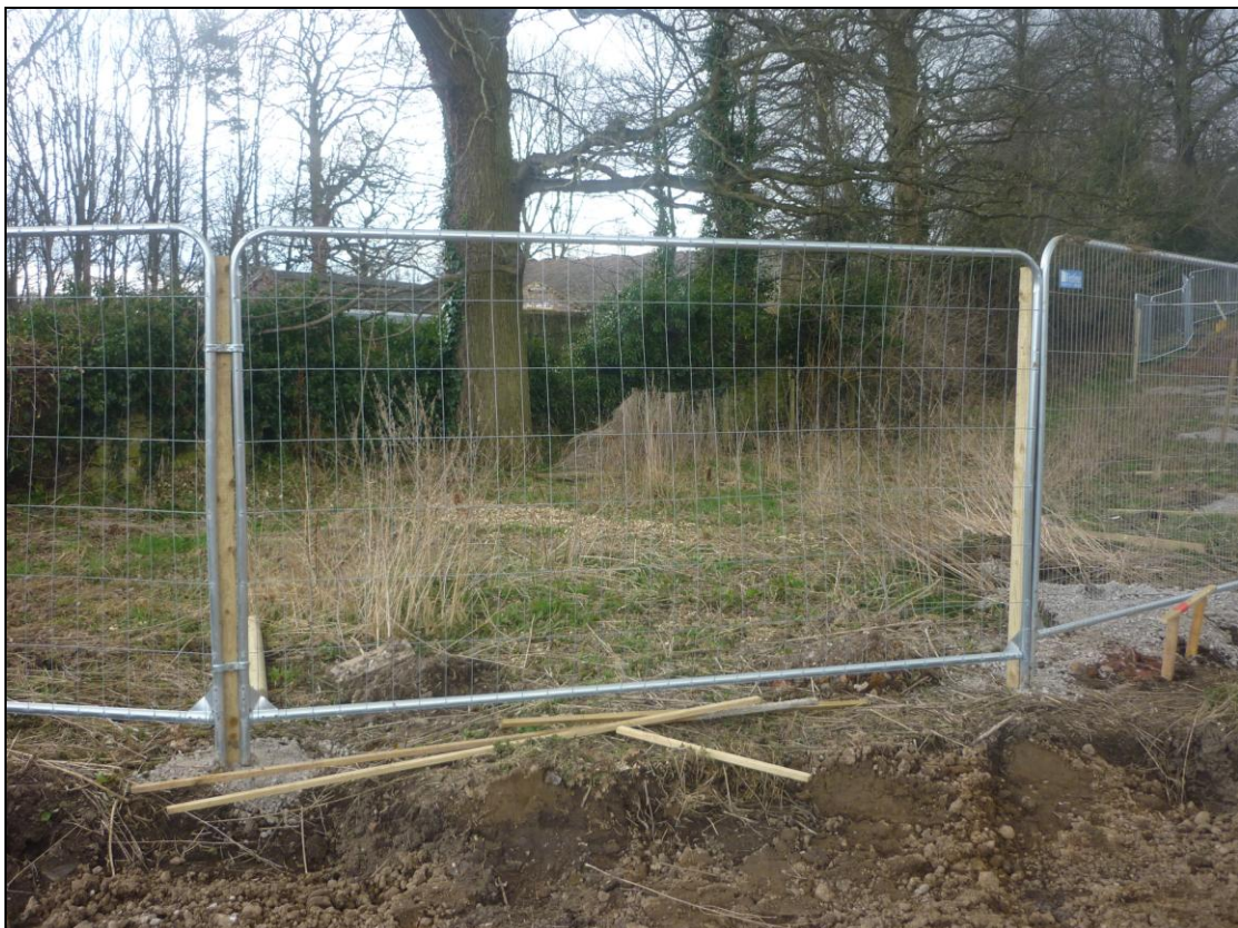
Photo 2 - Tree protective fencing erected to timber posts concreted in place to prevent movement
