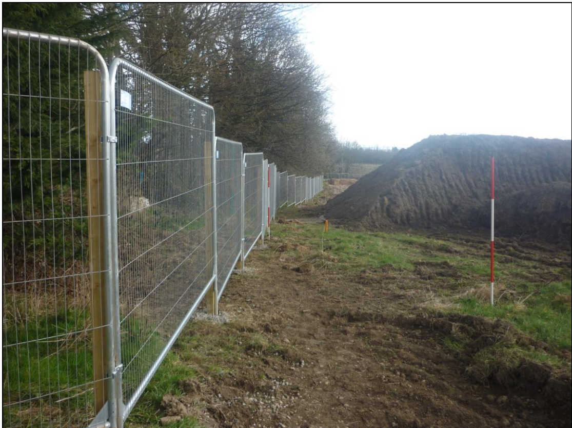
Photo 8 - Fencing erected along RPA of G4 & in accordance with approved Arboricultural Method Statement
