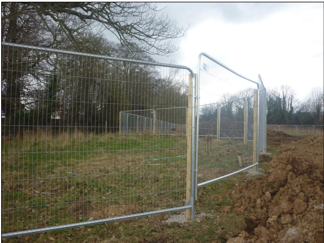
Photo 6 - Fencing around full extent of RPA of T3 & concreted in place to prevent movement
