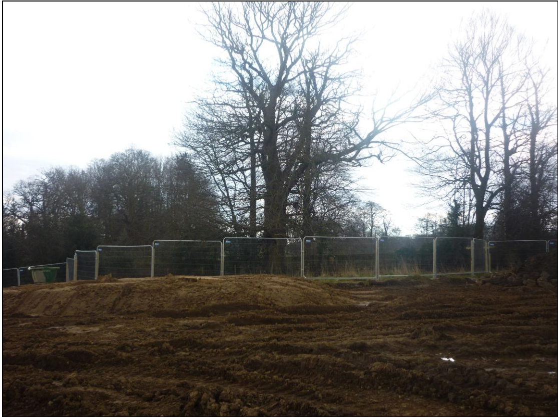
Photo 7 - Fencing around full extent of RPA of T3
