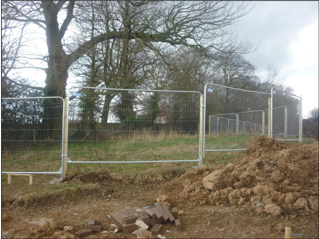
Photo 5 - Fencing around RPA of T3
