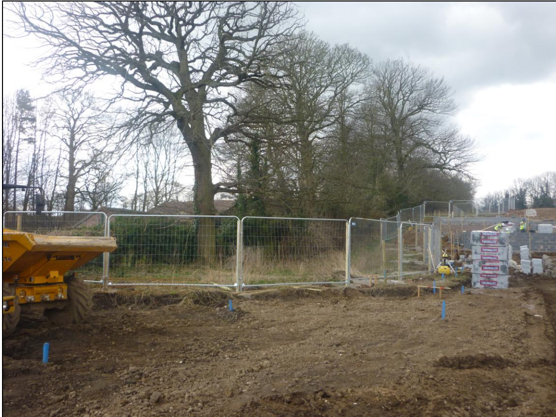
Photo 1 - Tree protective fencing erected to full extend of RPA of T1 & T2. Fencing will be realigned to secondary position and ground protection boards laid when scaffolding is due to be erected for plots 49 & 50
