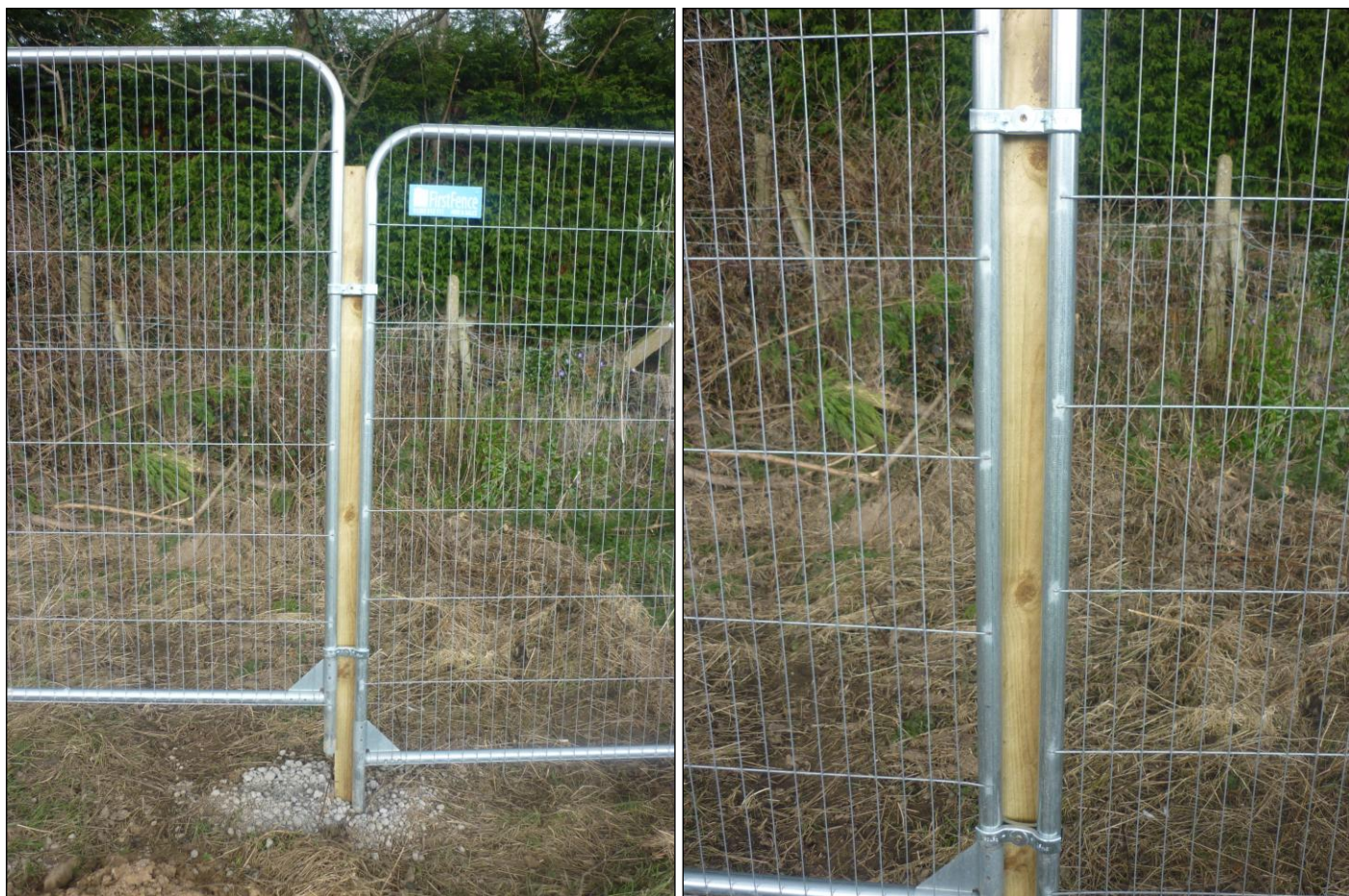
Photo 9/10 - Heras fence panels fixed to timber posts with ant-tamper bolts & post concreted into ground to prevent any movement during development works
