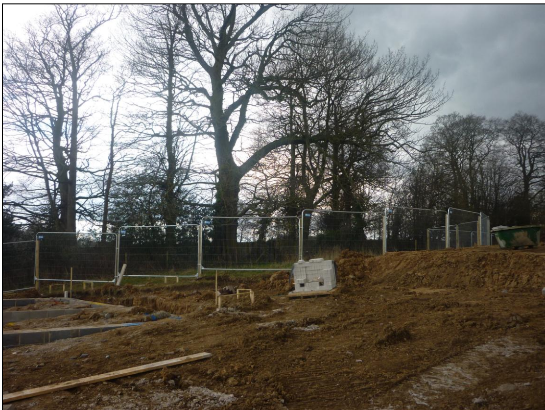
Photo 4 - Fencing in correct location around T3.
