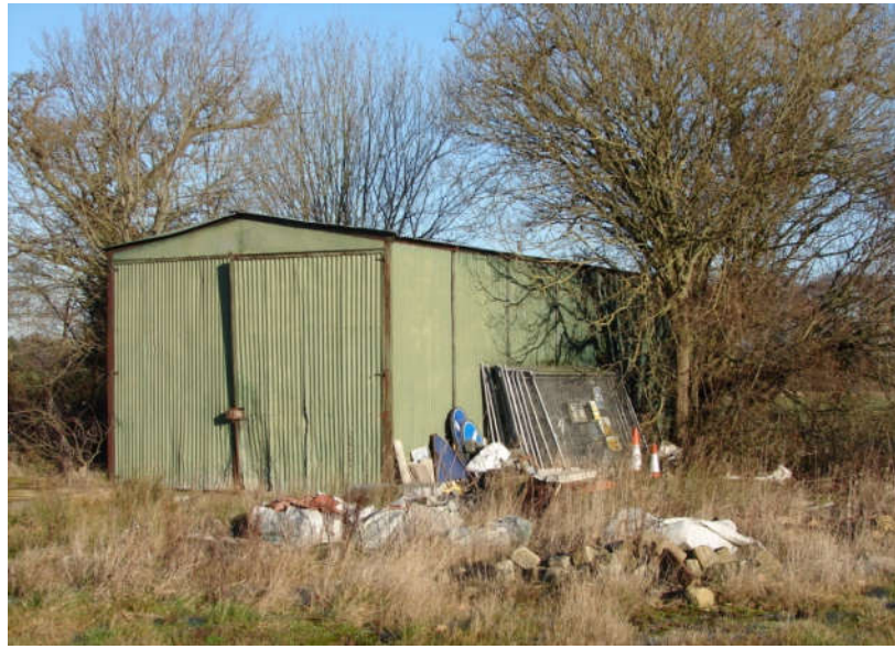
The building at Target Note 7 .
