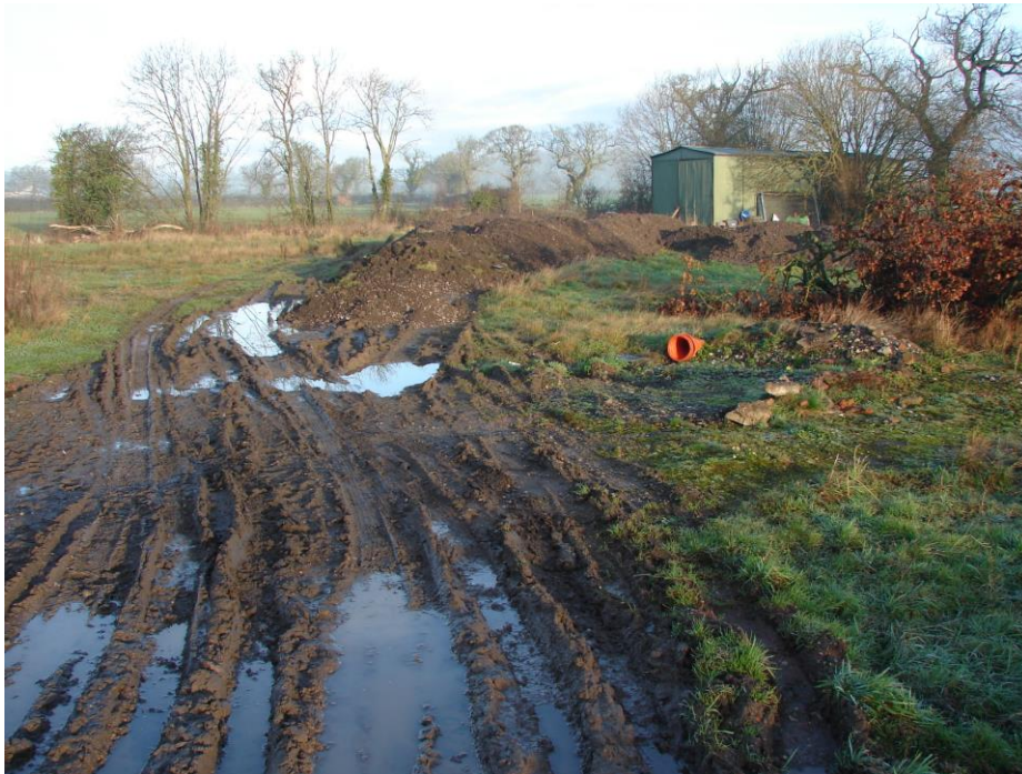
Piles of soil in the centre of the site and vehicle track.
