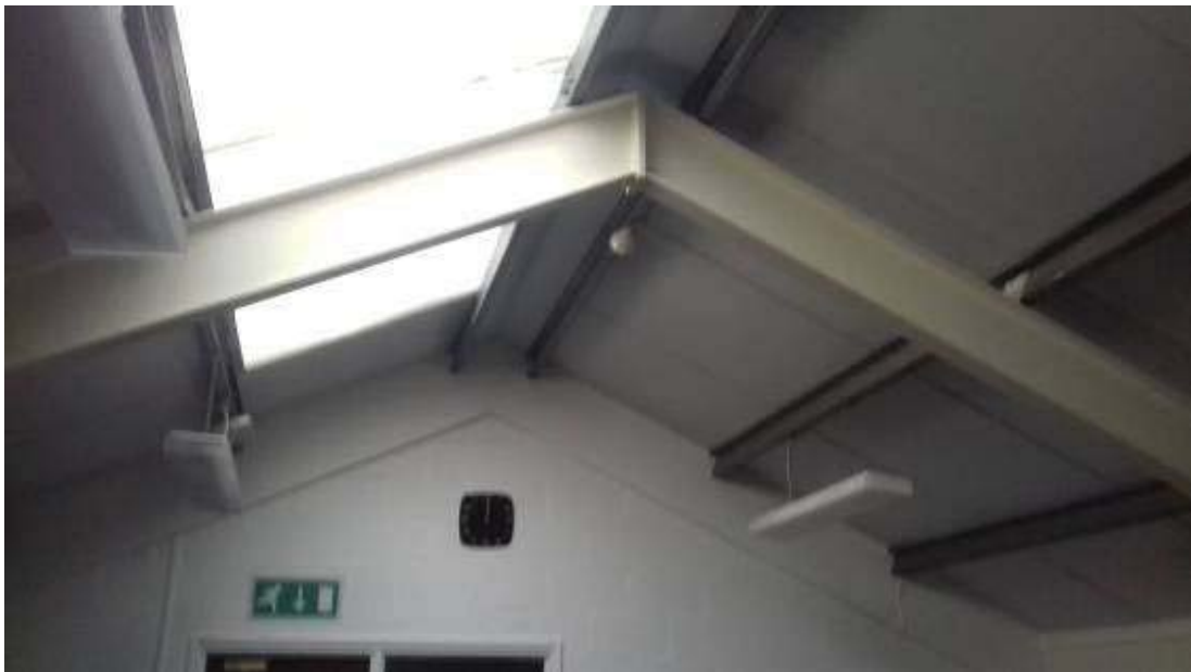
Plate 4: Area of B1 with vaulted ceiling
