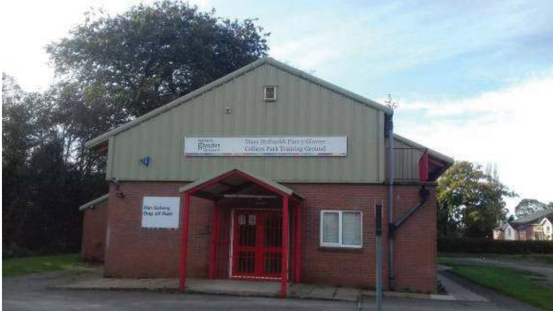
Plate 1: Front elevation of B1
