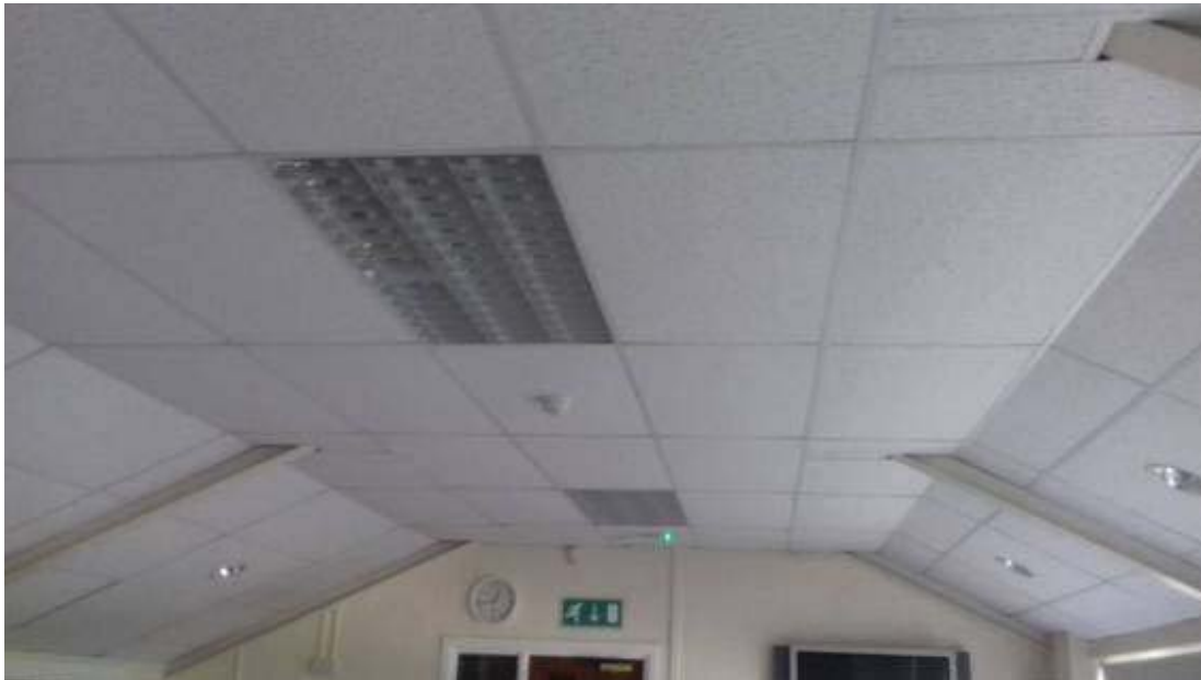
Plate 3: Interior section of B1 – vaulted ceiling with roof void above
