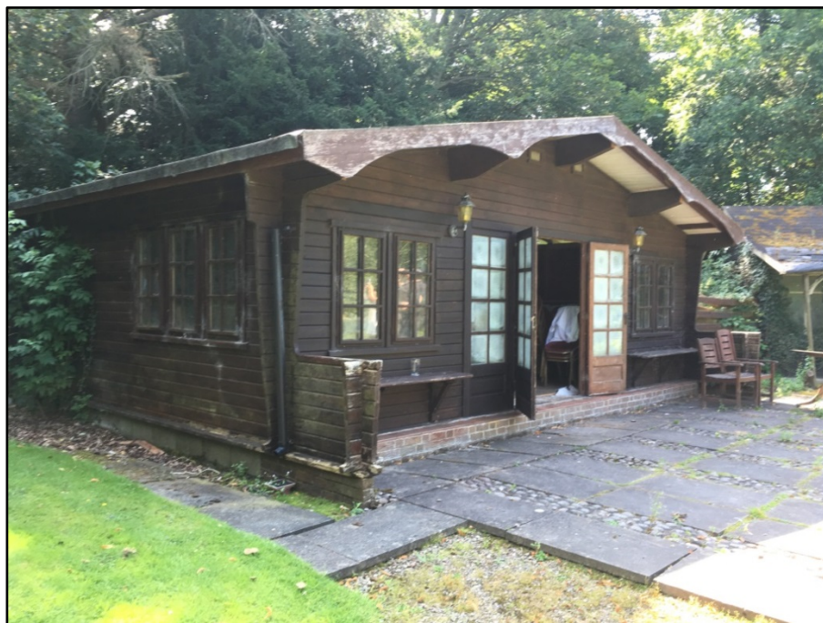
Figure 2 Existing wood cabins
