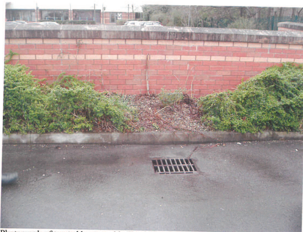
Photograph of treated knotweed in Total Fitness car park.
