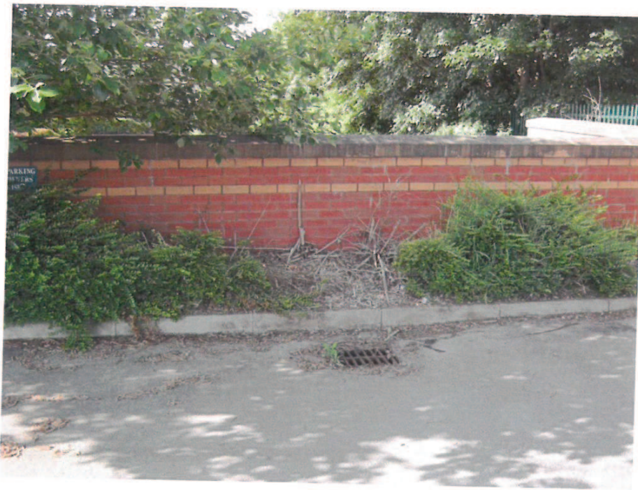
Figure A2.10 Looking south at small area of Japanese Knotweed behind the retaining wall
