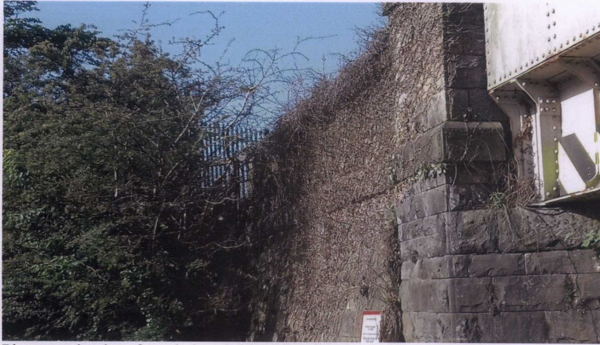
Photograph taken from below bridge showing fence line
