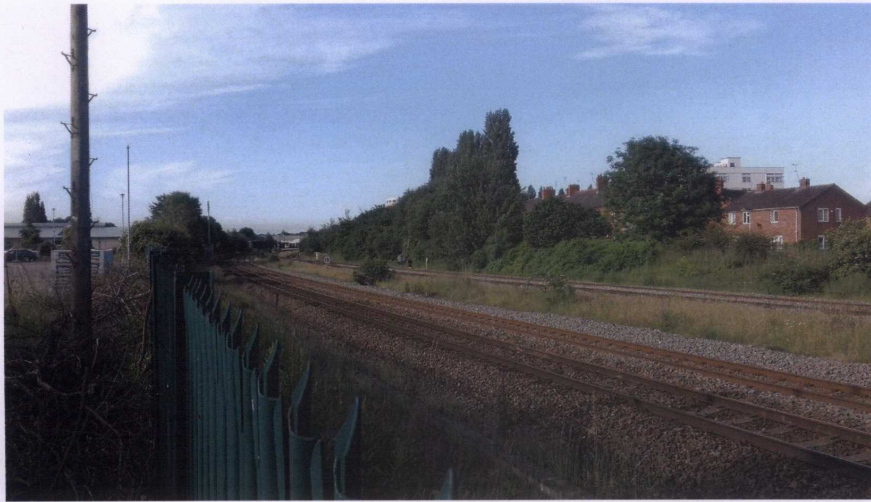
View looking south along the railway
