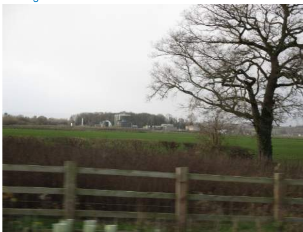
Photo E.27: View of the sewage works from the road, looking west
