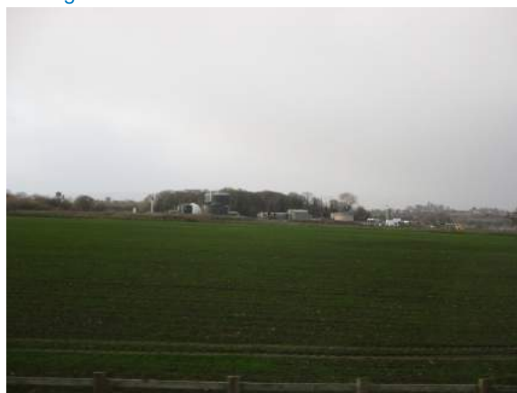
Photo E.28: View of the sewage works from the road, looking west
