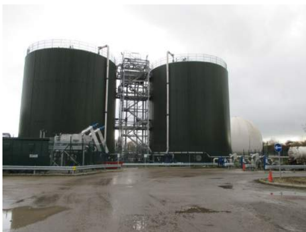
Photo E.7: Existing digesters, looking south
