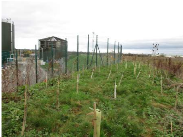
Photo E.17: Earth bank surrounding the southern section of the sewage works with sapling trees
