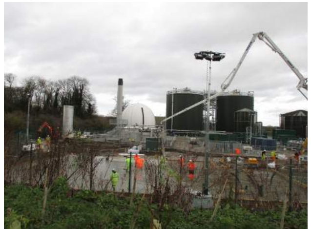
Photo E.20: Gas-to-grid plant construction taking place in the southern section of the treatment works (December 2014)
