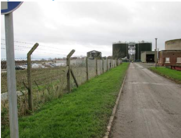
Photo E.3: Sewage structures including the existing digesters, looking south
