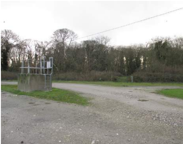
Photo E.35: Looking southeast towards the woodland from the path around the sewage plant
