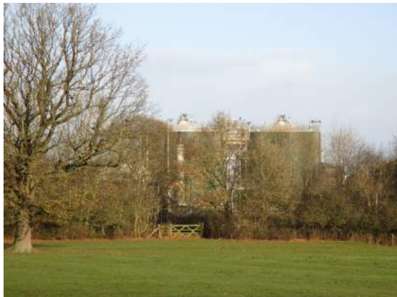
Photo E.45: Digesters looking north
