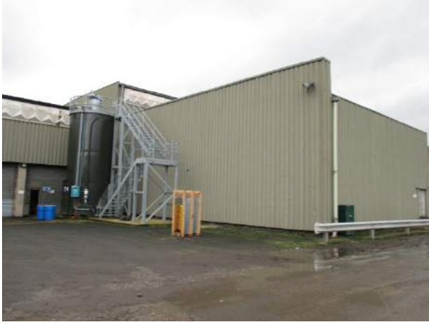
Photo E.9: Treated cake storage building containing asbestos
