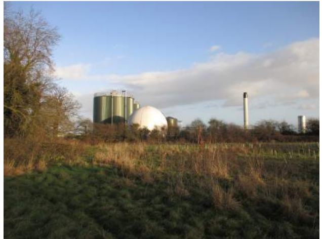
Photo E.30: Sewage treatment works, looking from an area of semi-improved grassland, located south of the broadleaved woodland
