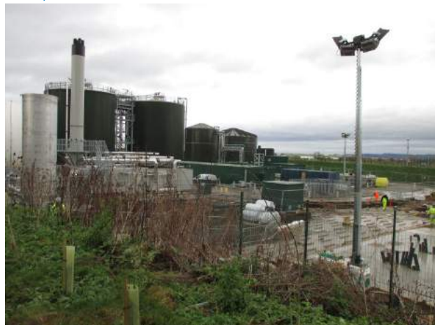
Photo E.22: Gas-to-grid plant construction taking place in the southern section of the treatment works (December 2014)
