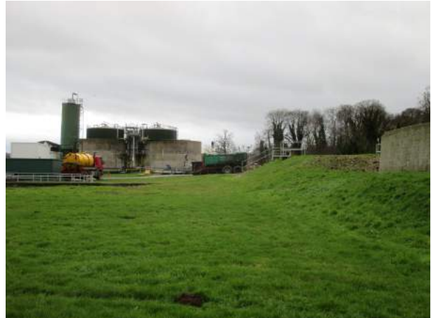
Photo E.2: Looking south, sewage structures including the lime silo, lime consolidation tanks, and digesters.
