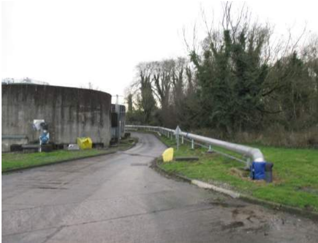
Photo E.39: Looking south towards the path east of the woodland and west of the disused sludge tank
