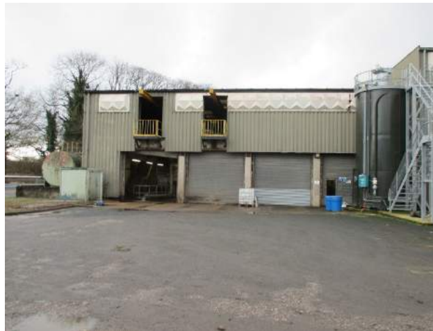
Photo E.6: Treated cake storage building containing asbestos
