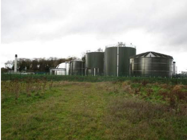
Photo E.13: Old sludge lagoon, looking west towards the sewage treatment works (including the screened sludge storage tank, digesters and the existing gas holder)
