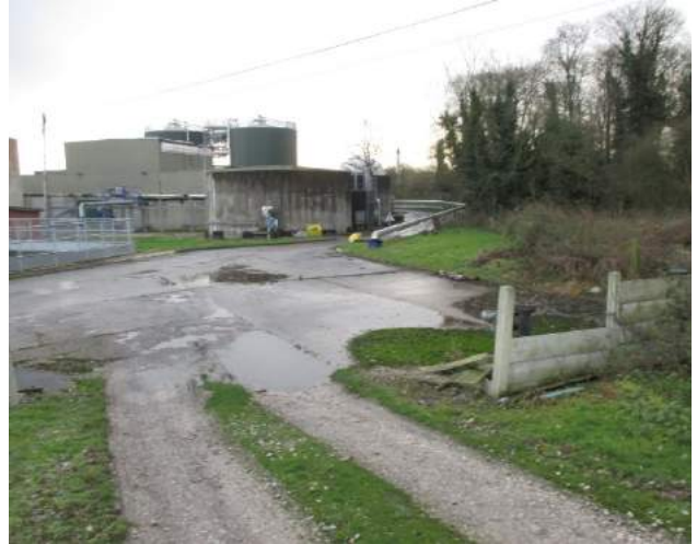
Photo E.38: Post digestion tank, disused sludge tank and the treated cake storage building adjacent to the ancient woodland
