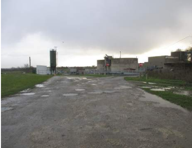
Photo E.37: Hardstanding area surrounding the sewage structures including the lime consolidation tanks, sludge holding tank, lime silo and treated cake storage building
