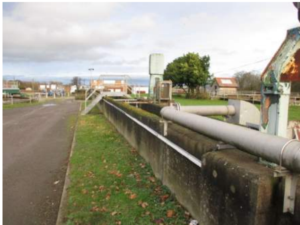
Photo E.25: Inlet channel for the F stream
