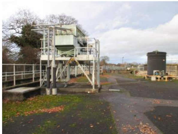
Photo E.26: Metal works structure adjacent to the inlet channel
