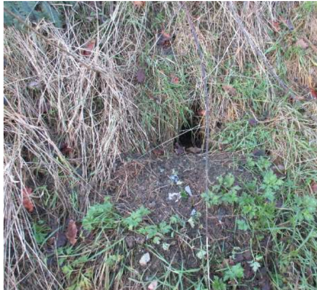
Photo E.70: A rabbit burrow within the earth bank surrounding the southern section of the sewage works
