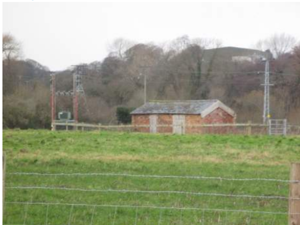
Figure E.77: A confirmed bat roost northeast of the sewage works
