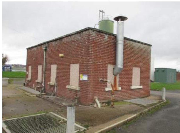
Photo E.4: Sludge Pump House building
