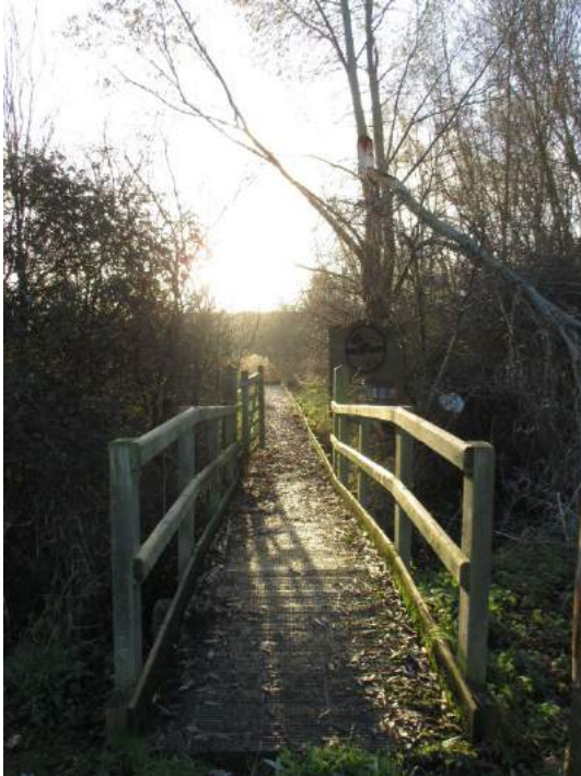
Photo E.49: Access bridge over a wet ditch into Marchwiel Marsh Nature Reserve
