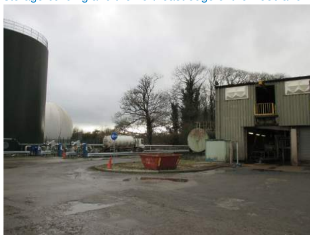
Photo E.8: Existing digester, gas holder, treated cake storage building and the northeast edge of the woodland
