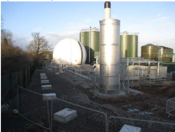
Photo E.31: Existing flare stack, gas holder and digesters, looking north from the earth bank
