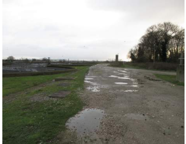
Photo E.34: Hardstanding path running around the unmanaged ancient woodland and sewage structures
