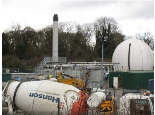
Photo E.18: Gas-to-grid plant construction taking place in the southern section of the treatment works (December 2014)
