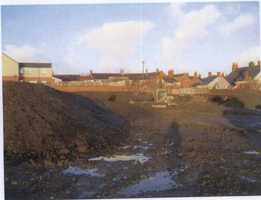
Photograph 8 Showing main section of site looking west
