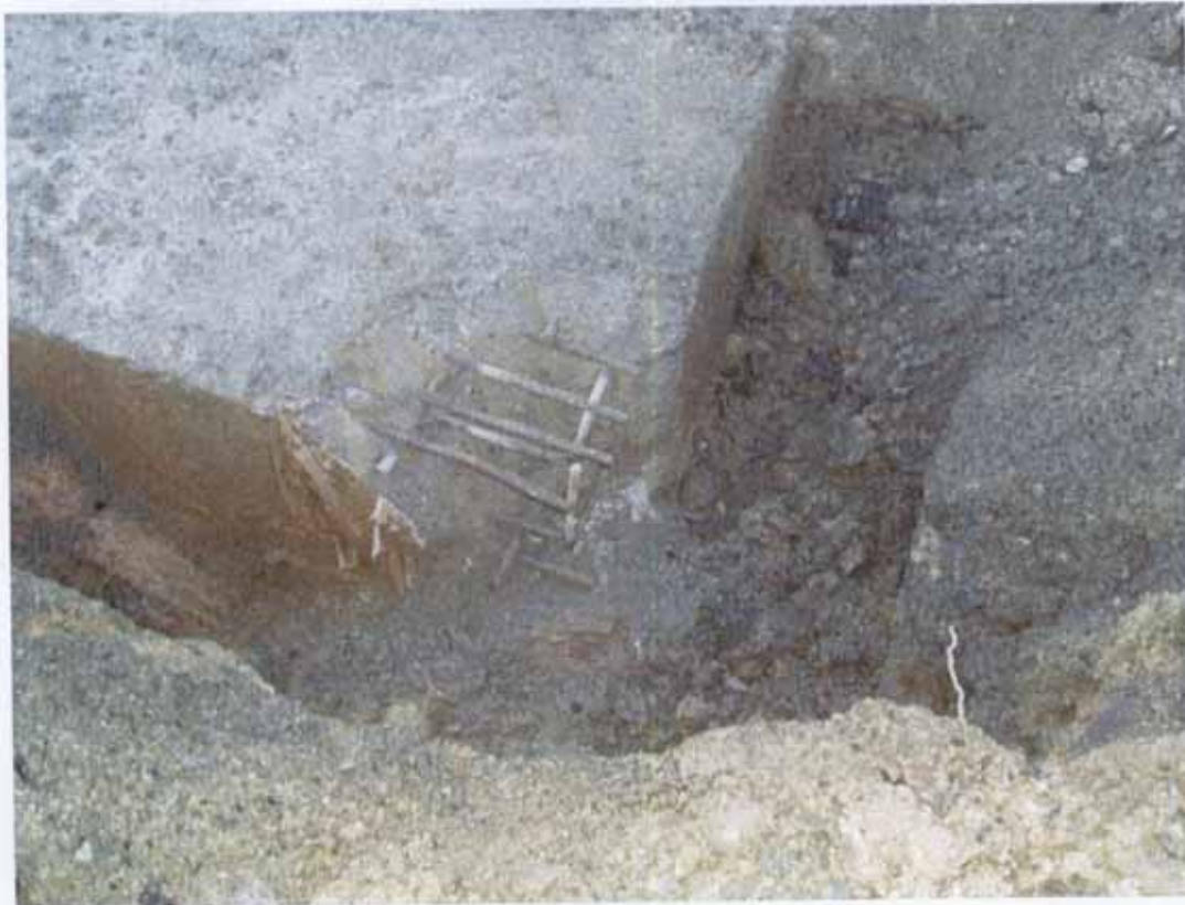
Photograph 5 Showing reinforcement in cap
