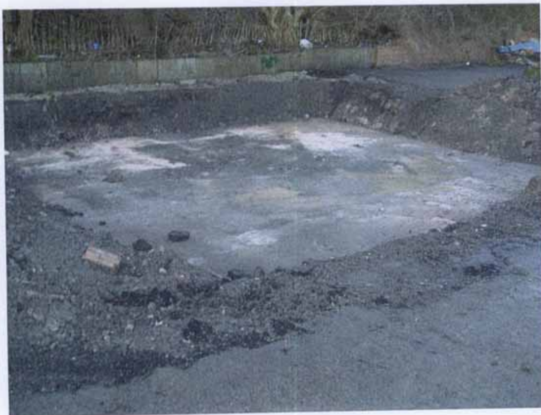
Photograph 6 Showing shaft cap
