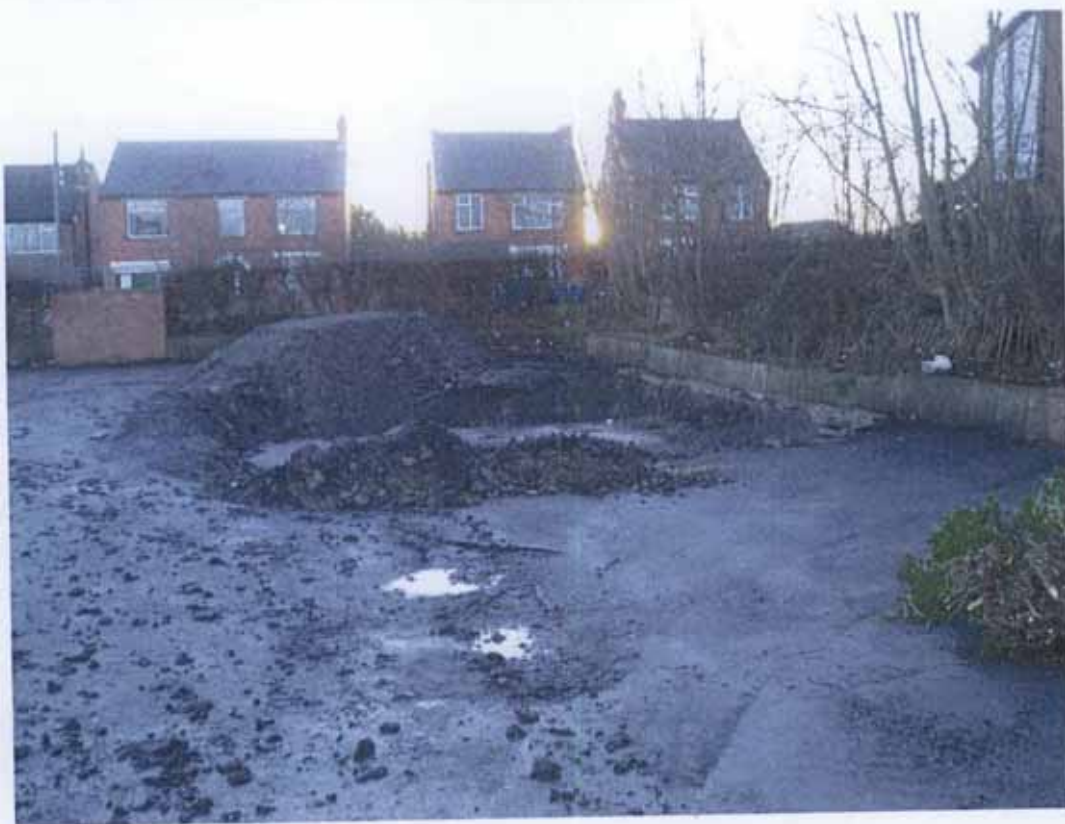
Photograph 4 showing shaft excavations on lower section of site
