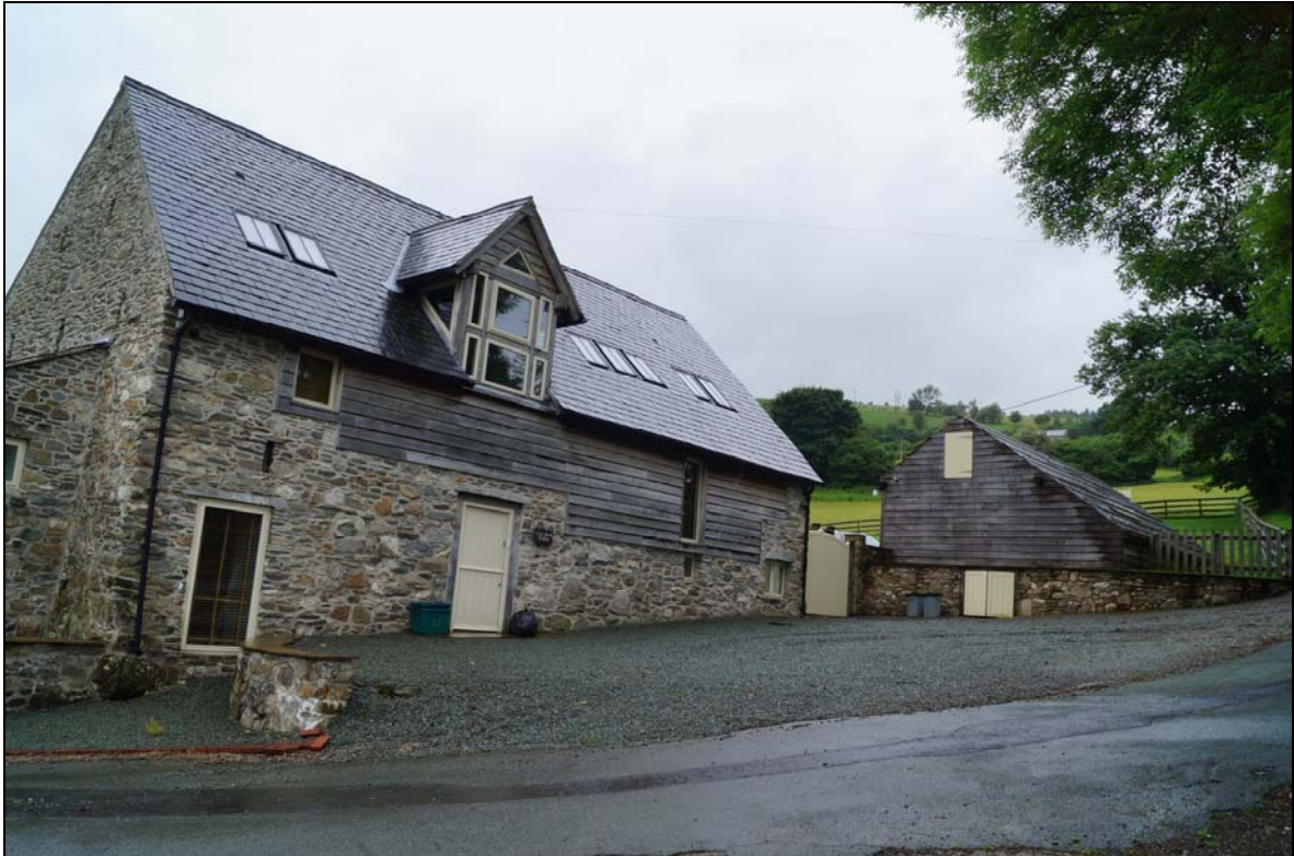
Plate 3: The listed barn at Cae Mor viewed looking south. The trees in the background would screen views of the proposed shed.
