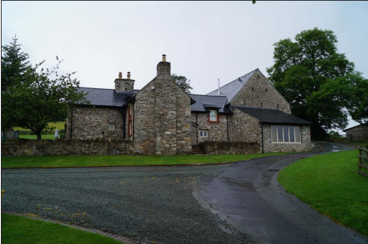
Plate 1: A key view of the farmhouse and barn at Cae Mor (ID number 4), looking west southwest from a minor road below the property. The house is to the left, the gable end of the barn to the right.
