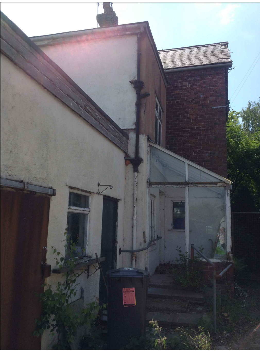
Existing Farmhouse - West Elevation
