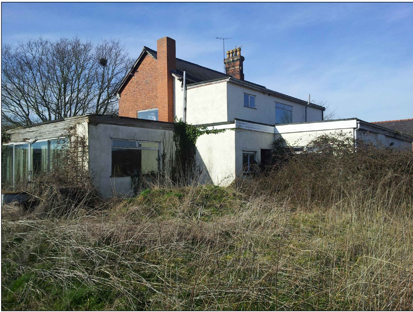
Existing Farmhouse - North Elevation
