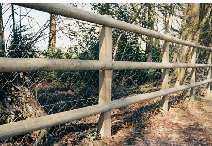
Timber Post and Rail (F6)
