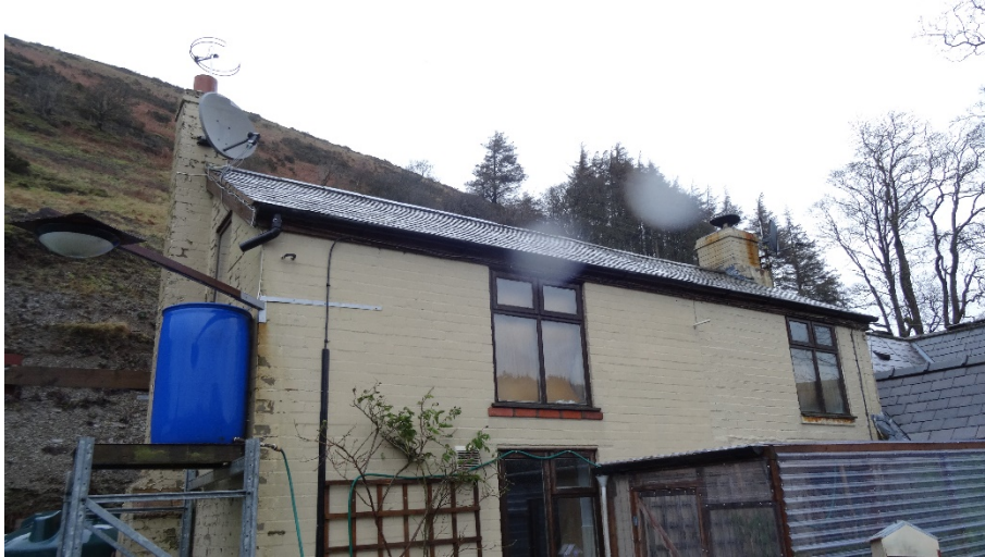
Figure 4. The double storey section to be retained, viewed from the south
