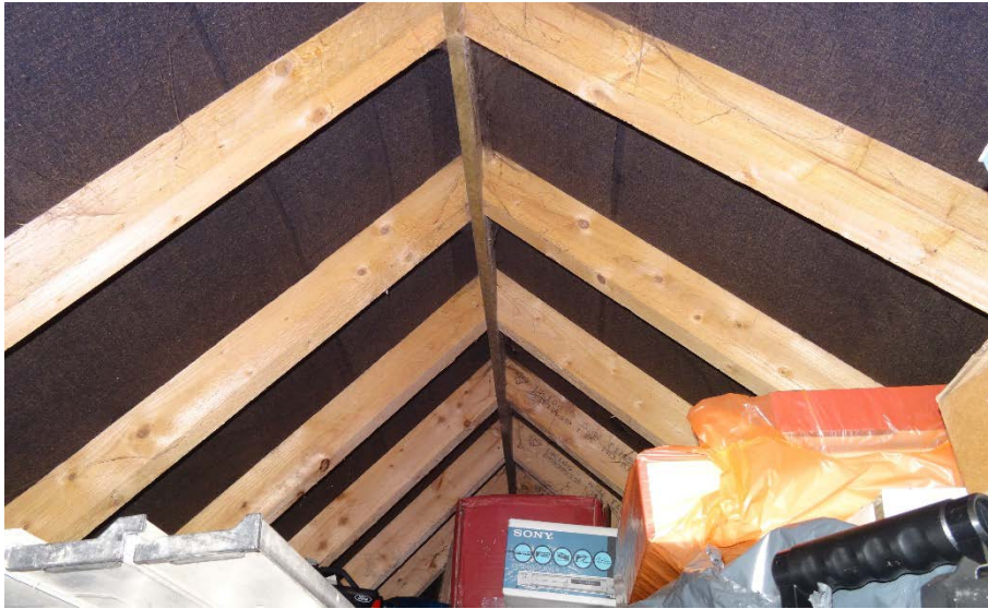
Figure 6. Inside the attic space of the single storey section of the dwelling
