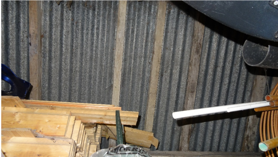
Figure 8. Inside the roof of the barn
