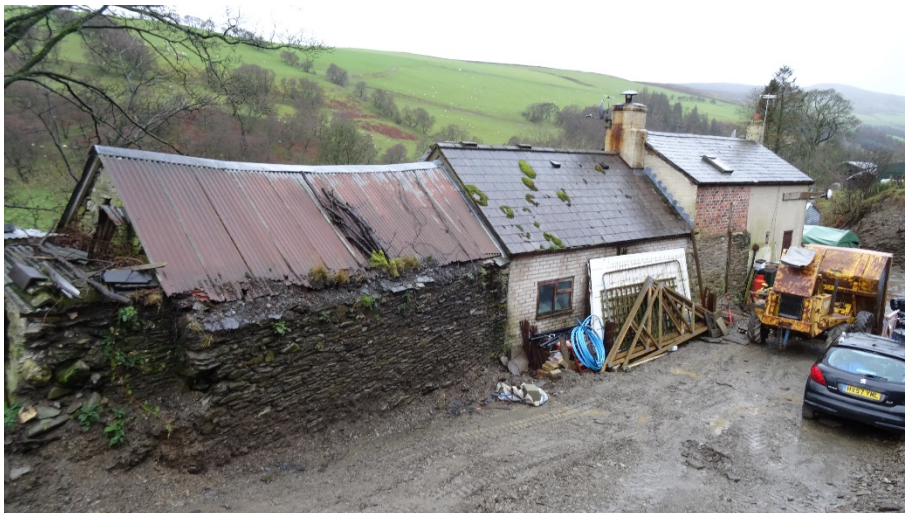
Figure 5. Showing the sections to be demolished, the rear of the section seen in Figure 4 is on the far right of this picture
