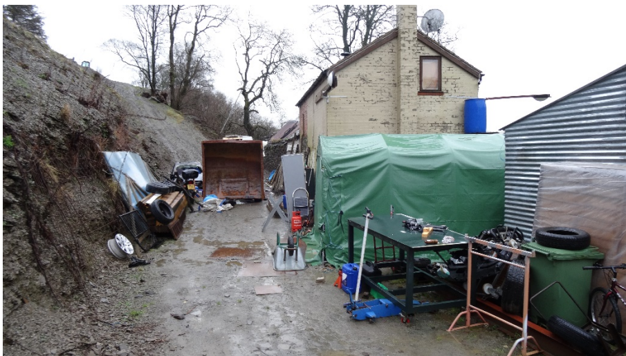
Figure 9. Showing the rear of the property, and the stone cut-out of the hillside on the left
