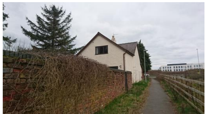
Croesnewydd cottage—Adjacent property to the site
