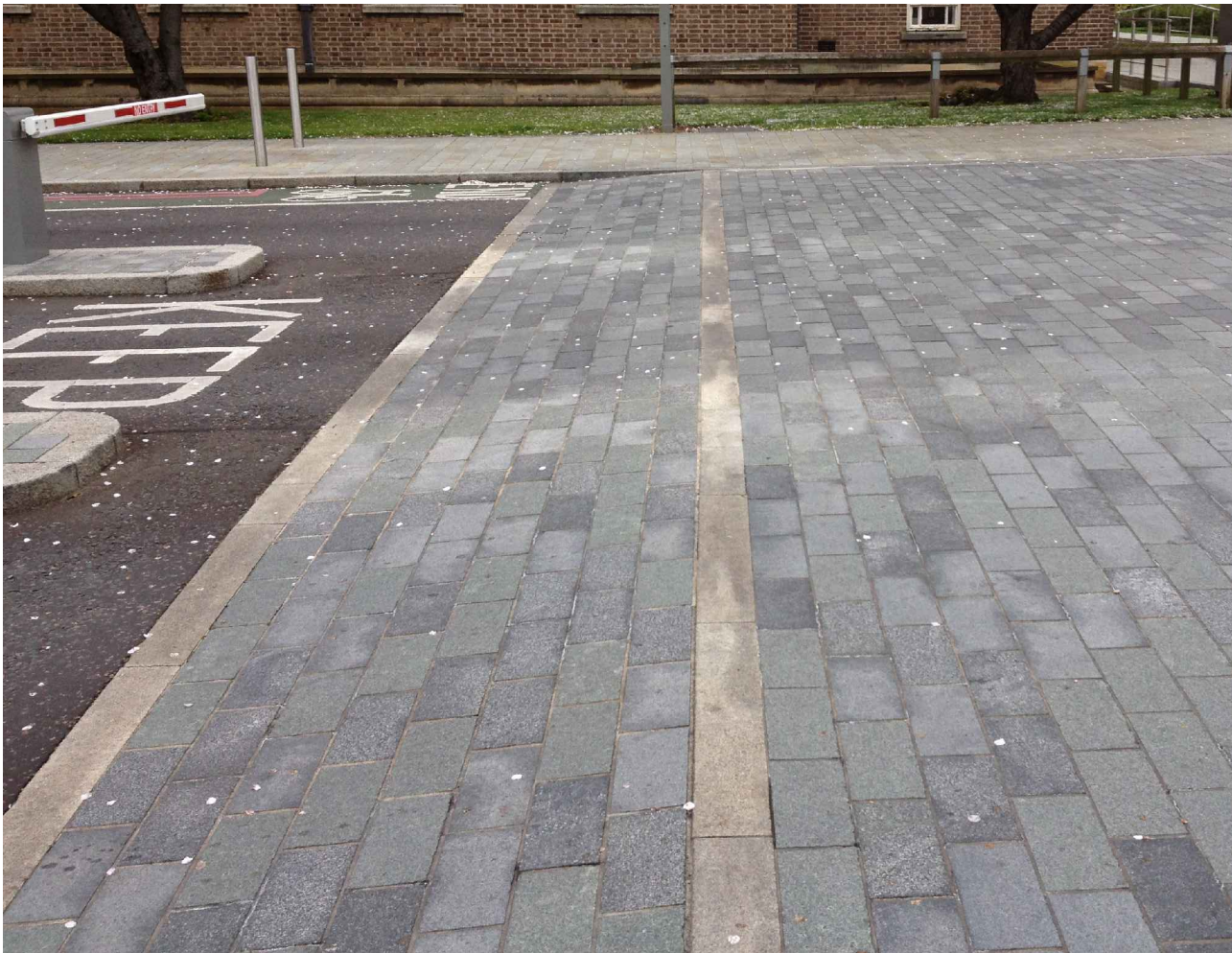
Raised carriageway tables across in unit paving
