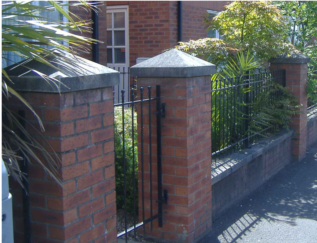
Brick Piers and Low Walls
