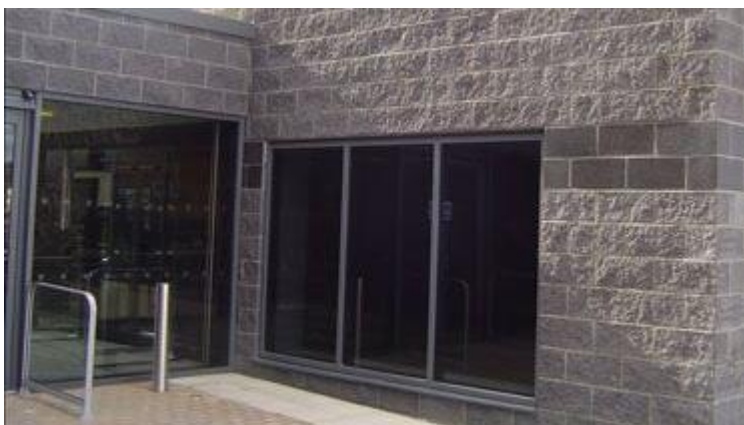
Example of blockwork plinth
