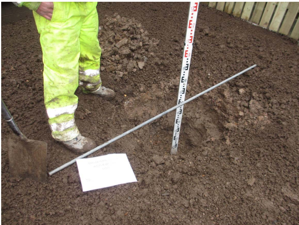
Photo 2 – Plot showing capping thickness >0.60m at Plot 9
