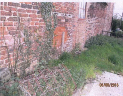
Figure 17: east side of barn
