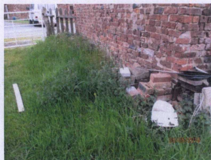
Figure 8: wall between end north compartment
