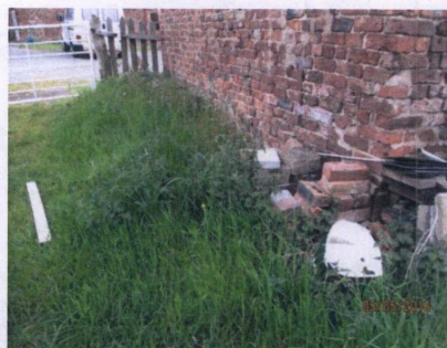
Figure 16: south edge of barn
