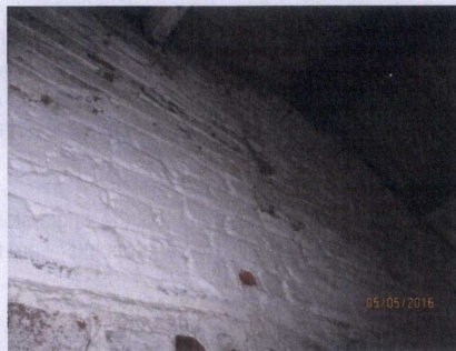
Figure 6: entire wall, Compartment 2
