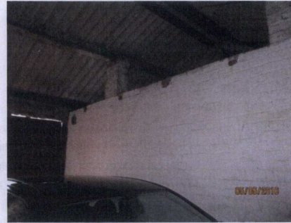
Figure 5: partial internal brick walls
