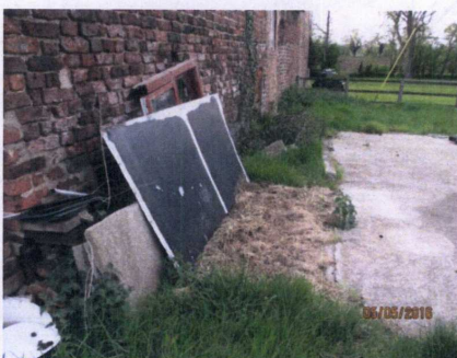
Figure 15: east side of barn
