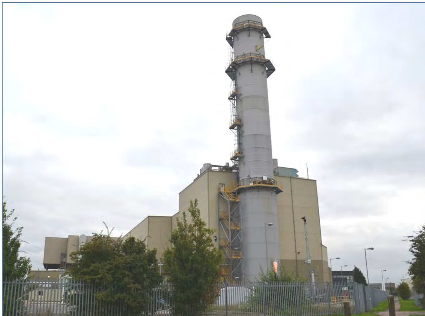
Figure DAS25: View of a typical operational HRSG and Stack. (For illustrative / explanatory purposes only.)
