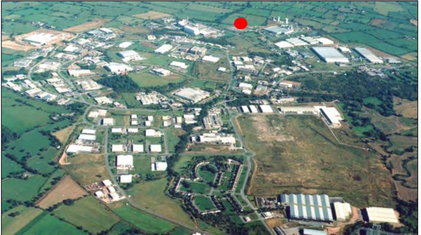
Figure DAS3: aerial photograph of the WIE. Looking north-east, circa 1990s, with the Power Station Complex site identified. Source: WPL
