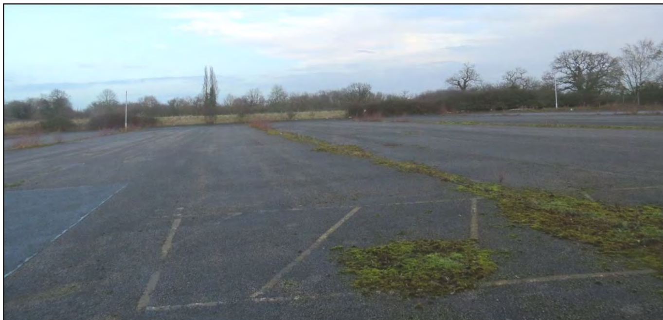
Figure DAS09: View from the southern boundary across the hardstanding area January 2015.
