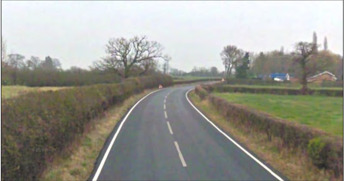
Figure DAS33: Oak Road, close to position of Gas Connection Route. Looking SW towards Ourholme.
