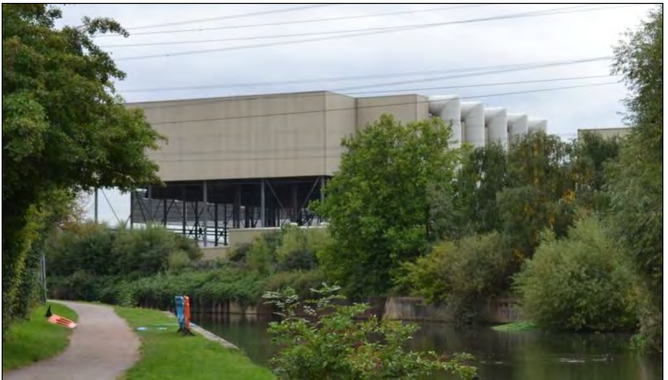
Figure DAS26: Exterior of an air-cooled condenser for a power station. Enfield Energy Centre: For illustrative purposes only
