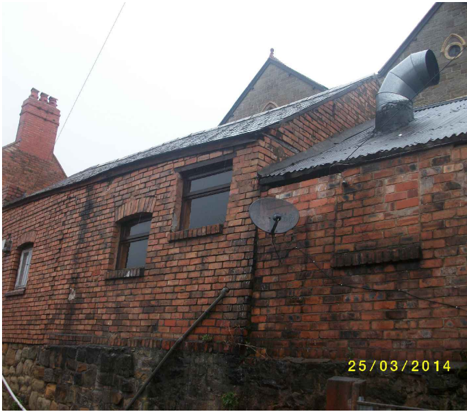
Existing Apperance of Rear Walling Repointing Sample panel requires approval
