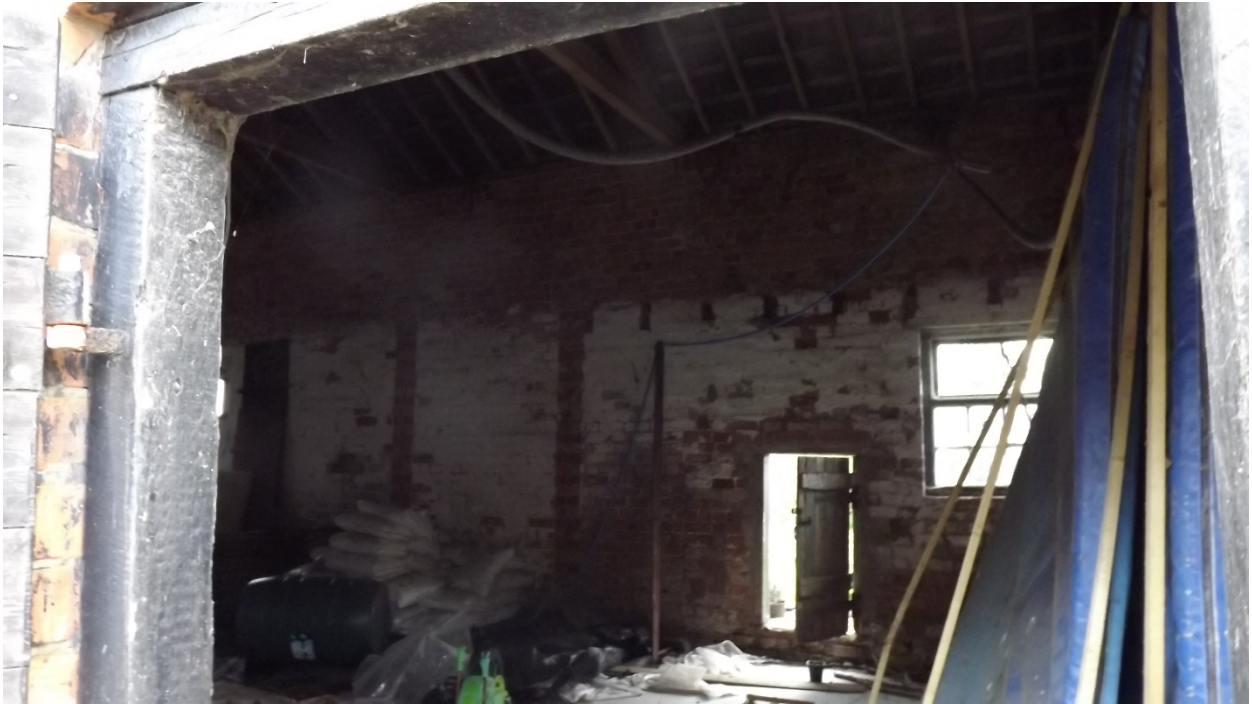
Figure 9. Showing the interior of the eastern end of the south building.
