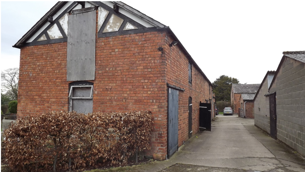
Figure 7. Looking west, showing the south building (pictured on the left)
