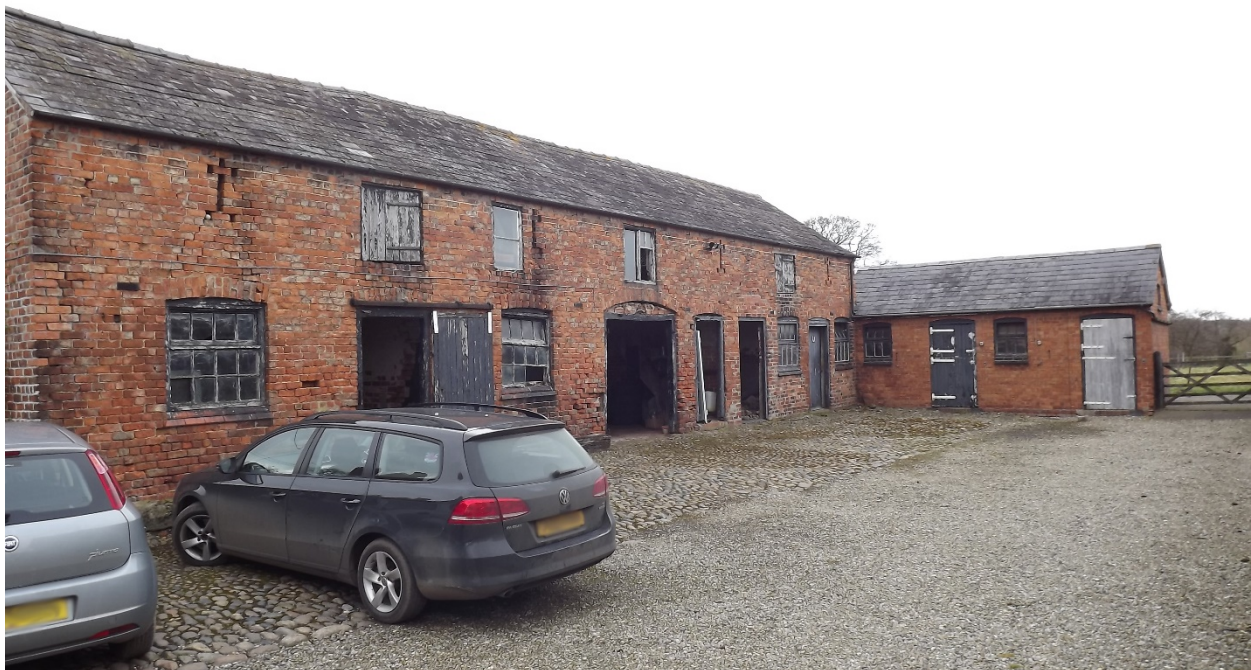
Figure 4. Looking north at the north building. The small building to the right of the image is the pig pen
