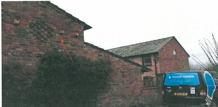
North facing elevation on which bird boxes are present
