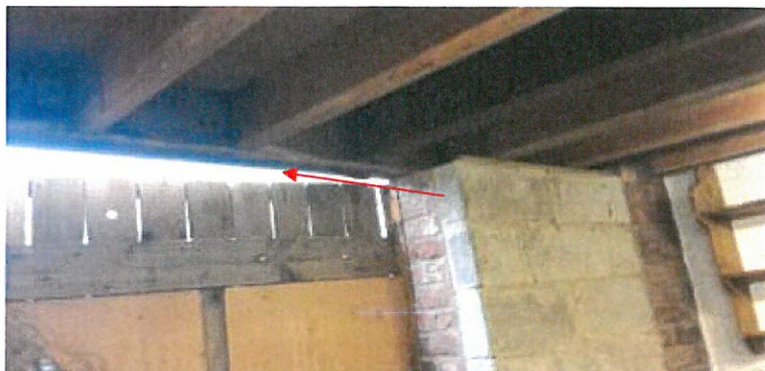
Access opportunity typical of those throughout which would be utilised by nesting birds
