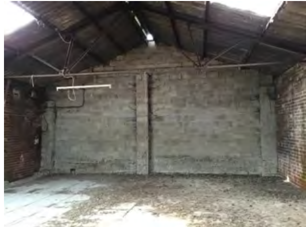
Blockwork partition wall built to separate the barn into two rooms.
