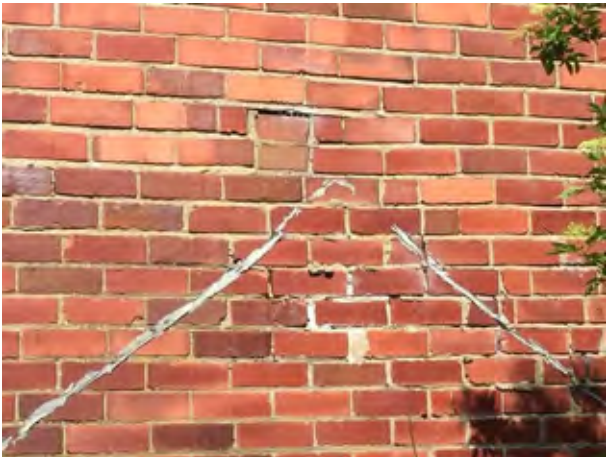
Masonry moved inwards where previous roof structure abutted the elevation.
