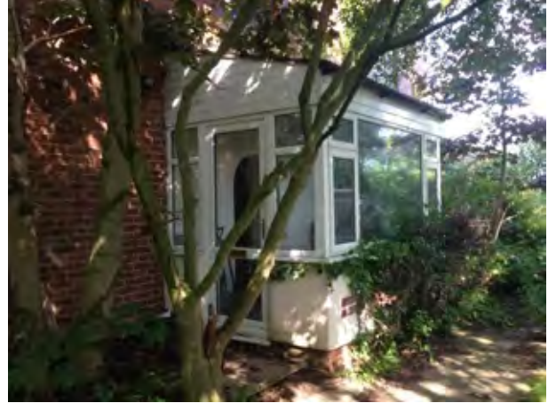
Porch structure. Trees close to front elevation.
