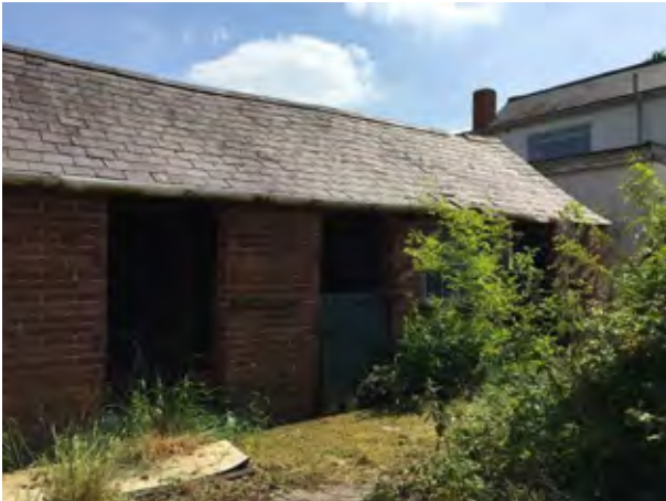
Right hand side of front elevation.
