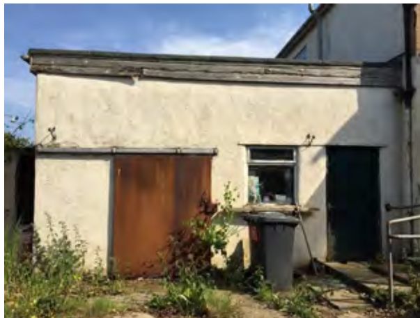
Left hand side of single storey extension at the rear of the property.
