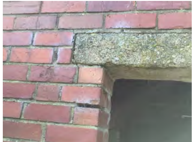
Movement of brickwork to bearing for lintel.
