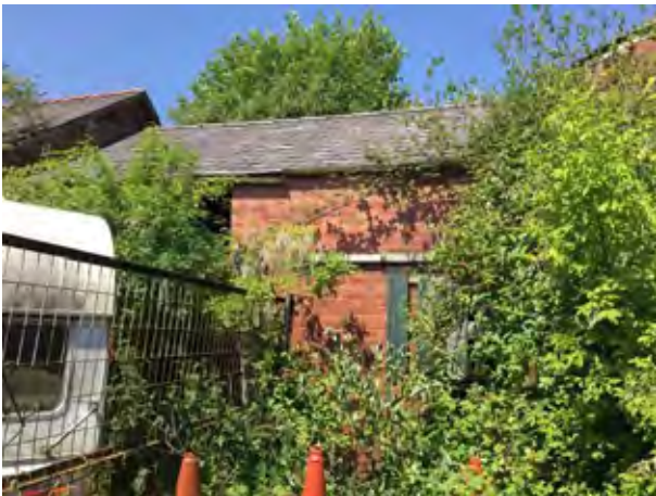
Extended part of barn hidden by vegetation
