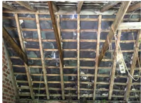
Existing ties across roof. Hole through roof.
