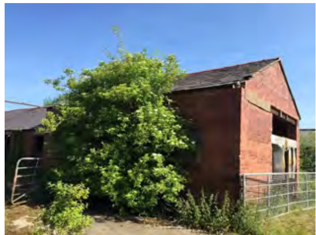
Front elevation of the two storey part of the barn.
