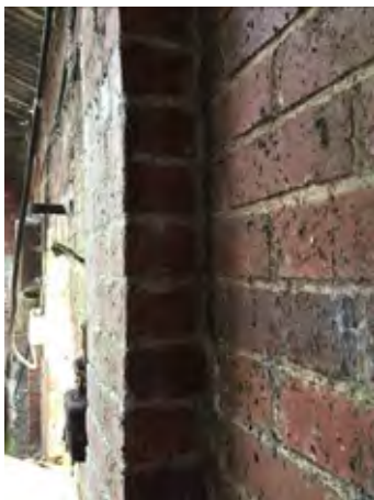
Brick pier on rear wall.
