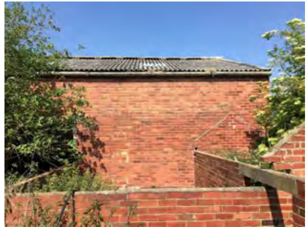
Left hand side of rear elevation.
