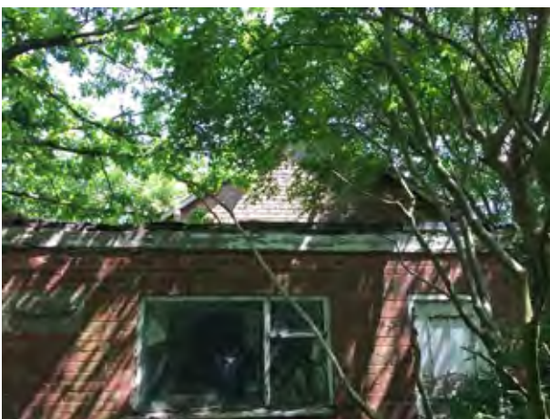
Single storey structure in front of elevation.
