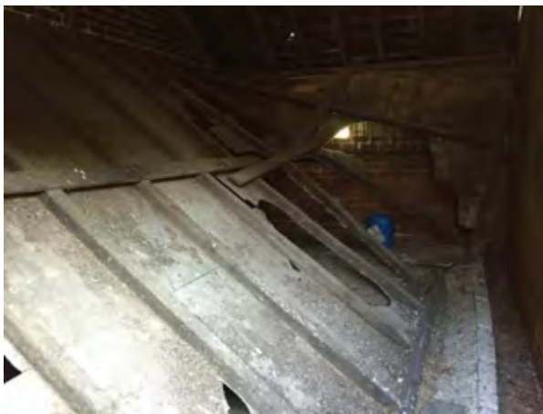
Collapsed ceilings.
