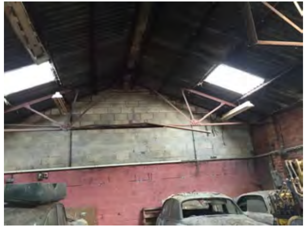
Blockwork partition wall between Room 1 and 2.
