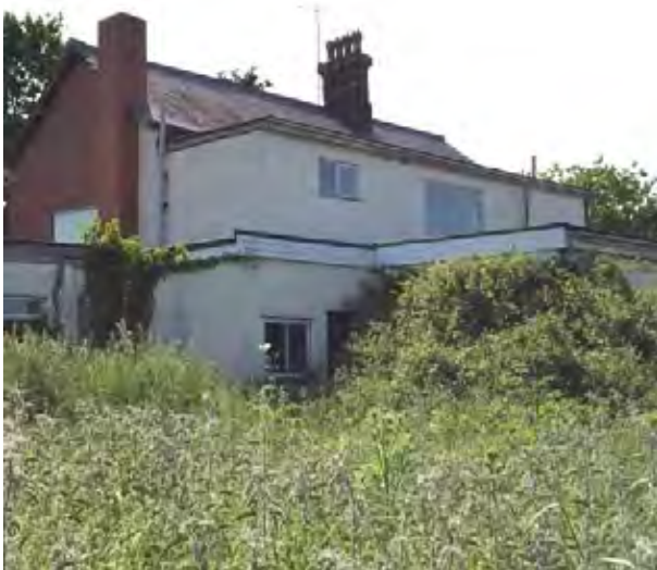
Rear elevation generally.
