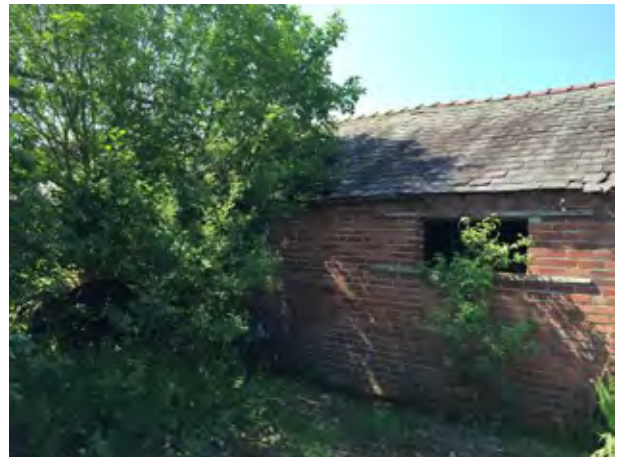
Undulating roof to rear elevation.
