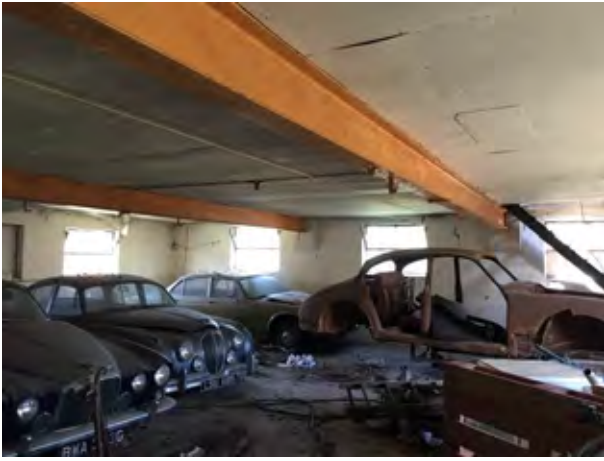
Steel beams supporting the first floors.
