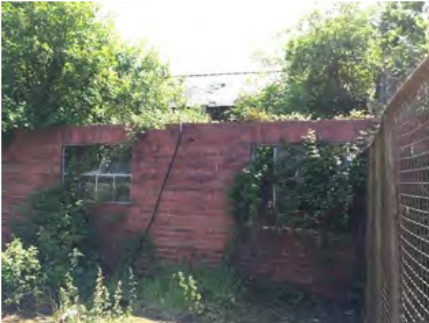
Structure in front of rear elevation.
