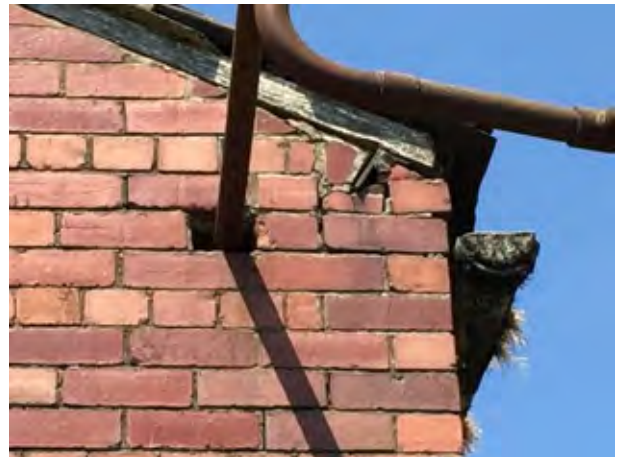
Holes through elevation for pipework.
