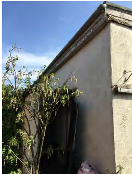
Rear of single storey rear extension.
