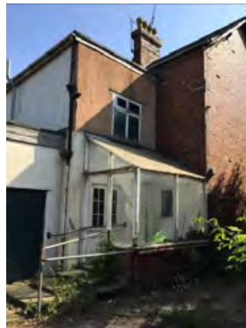
Rear porch on left hand side elevation.
