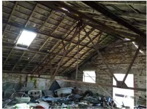
Steel truss supporting roof structure.
