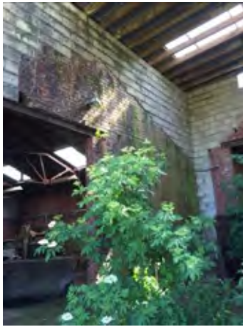
Large opening from through the right hand side gable wall. Blockwork constructed over original gable profile to increase height of adjacent barn.
