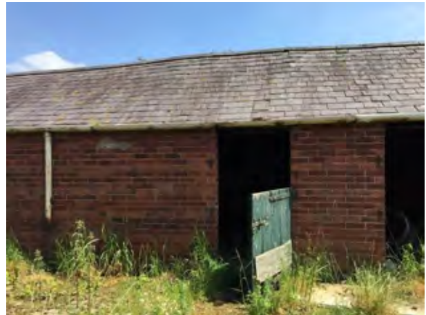
Central area of front elevation.
