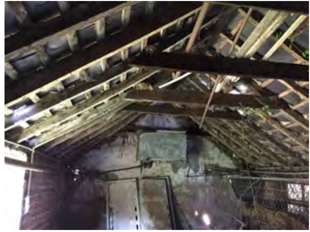
Typical roof configuration.
