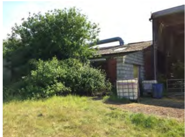
Right hand side of front elevation.
