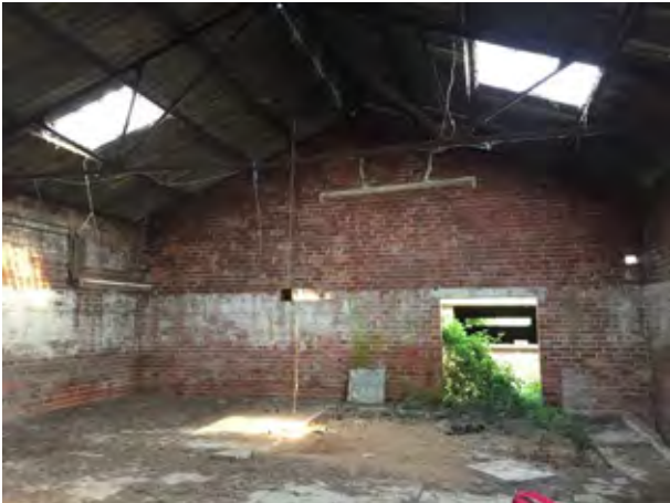
Internal face of left hand side elevation.
