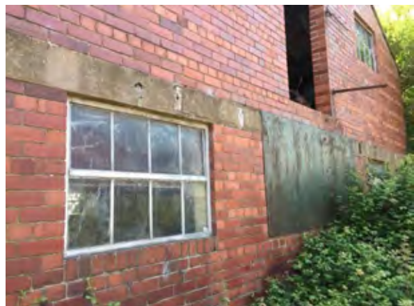
Concrete ring beam with timbers built in.
