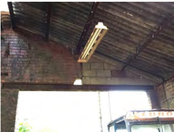
Steelwork installed to form large opening/
