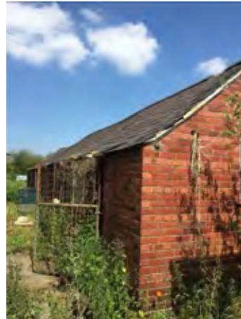
Undulating roof slope.
