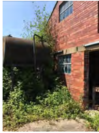
Tank and vegetation hiding elevation to right hand side.
