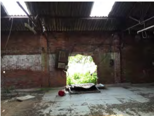
Large opening formed through rear wall.
