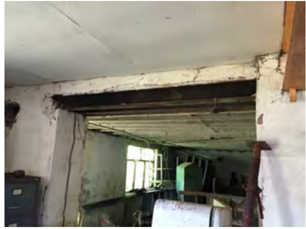
Steel beams forming the opening between Barns 1 and 2.
