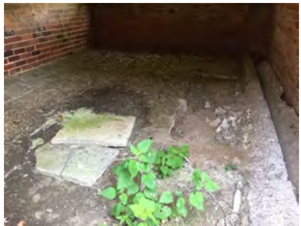
Concrete paving slabs and trough noted.
