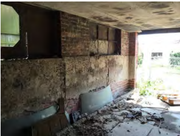
Internal area at ground floor level with the two storey part of the barn.
