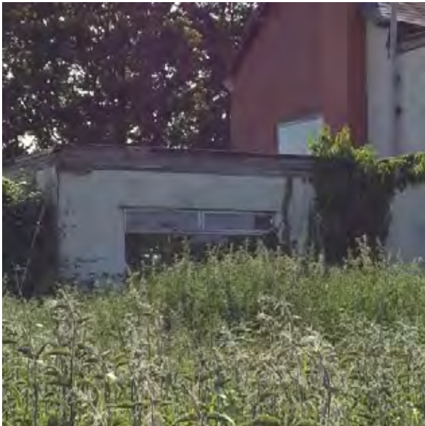
Rear elevation of side extension
