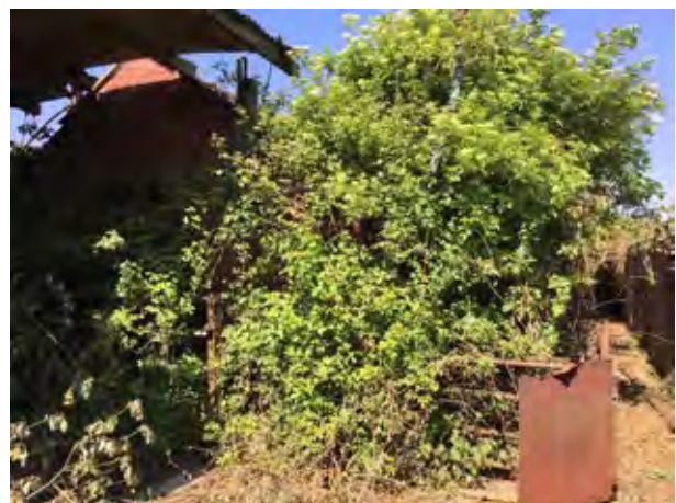
Majority of the elevation is hidden by vegetation.
