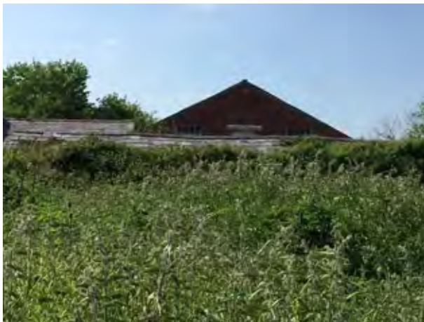
Rear elevation hidden by vegetation. Close access not available.
