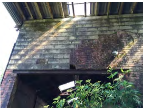
Large opening from through the right hand side gable wall. Blockwork constructed over original gable profile to increase height of adjacent barn.
