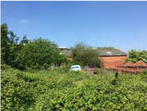
Rear elevation hidden by trees and vegetation.
