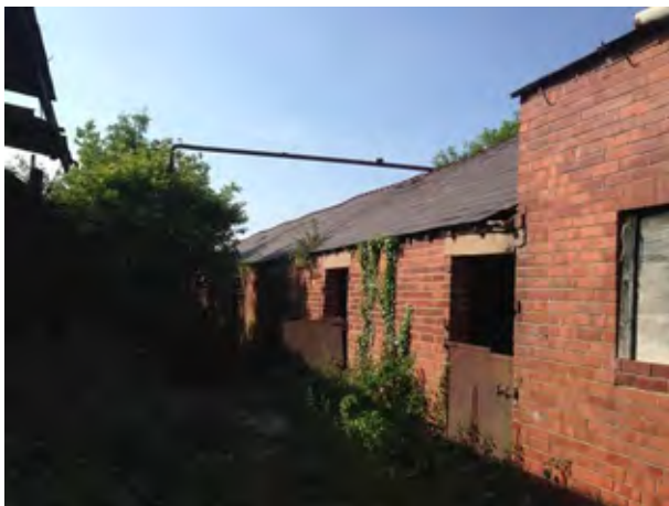
Front elevation of single storey part of the barn.
