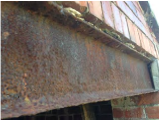
Corroding steelwork.
