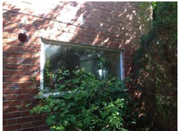
Large window opening at ground floor level.
