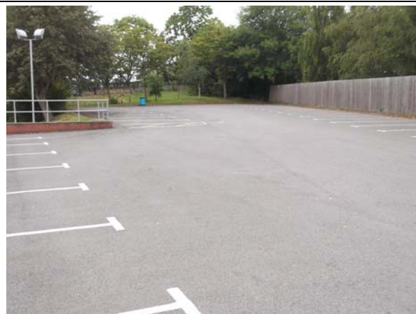
Photograph 8 – Hard-standing parking areas
