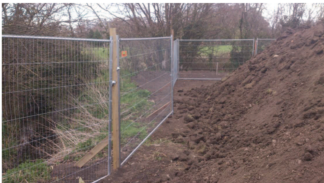
Photo 3 - Weldmesh tree protective fencing in place around G1 & T3
