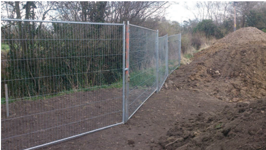
Photo 5 - Weldmesh tree protective fencing in place around G1
