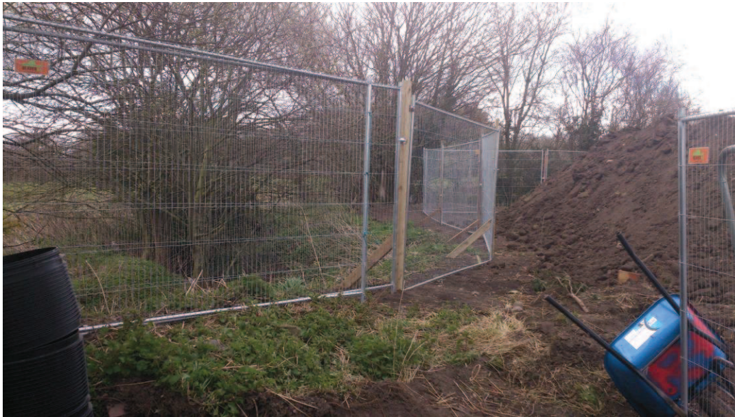
Photo 4 - Weldmesh tree protective fencing in place around G1 & T3
