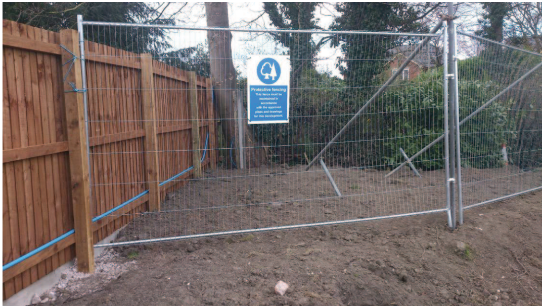
Photos 1 – Weldmesh tree protective fencing in place around tree number 1
