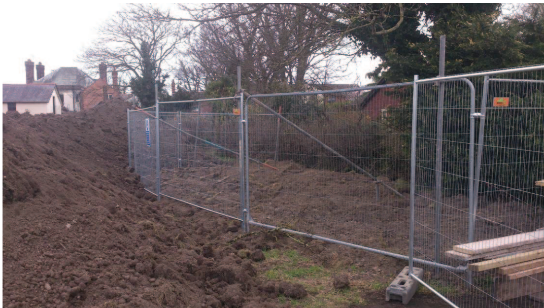
Photo 2 - Weldmesh tree protective fencing in place around tree number 3
