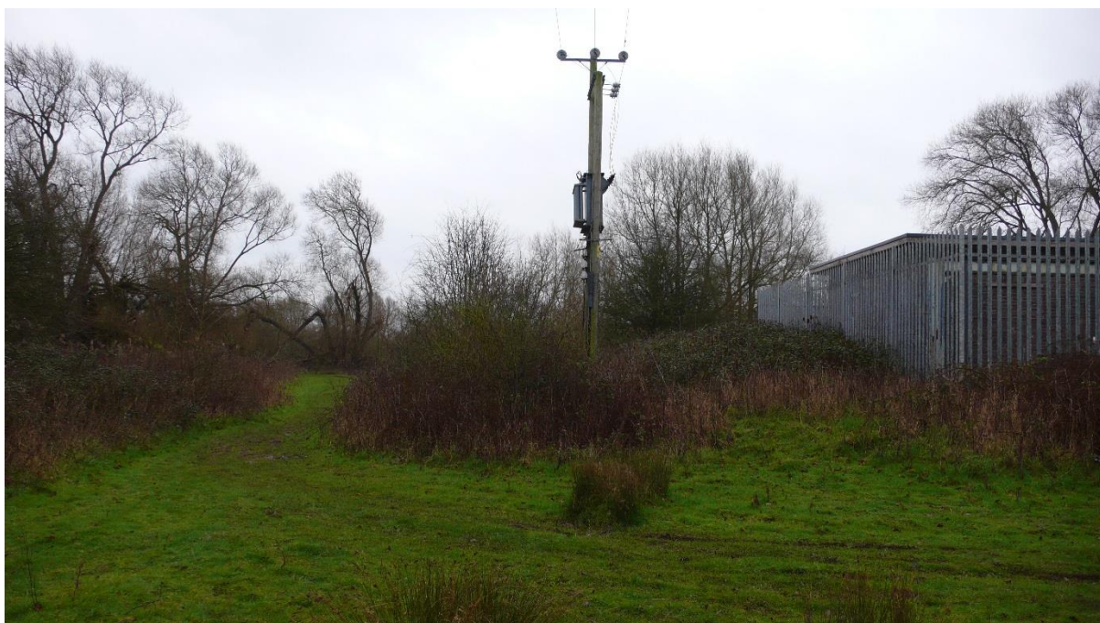
Pole 2 to be replaced by Pumping Station
