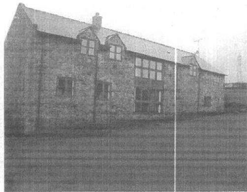
Figure 1: The north elevation
