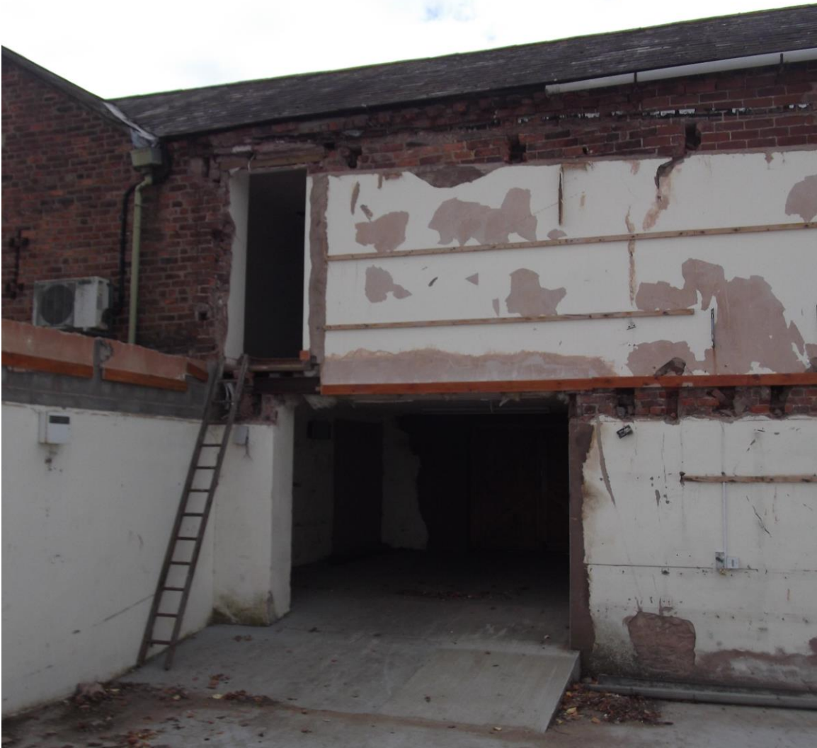
Picture 9 Door at first floor level on rear elevation
