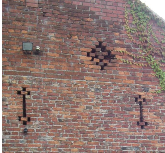
Picture 5 Brickwork details on external walls
