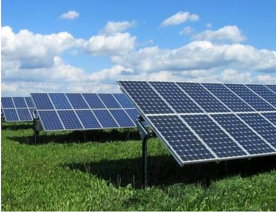
Frame mounted solar panels – the illustration shows a "2 portrait" arrangement.
