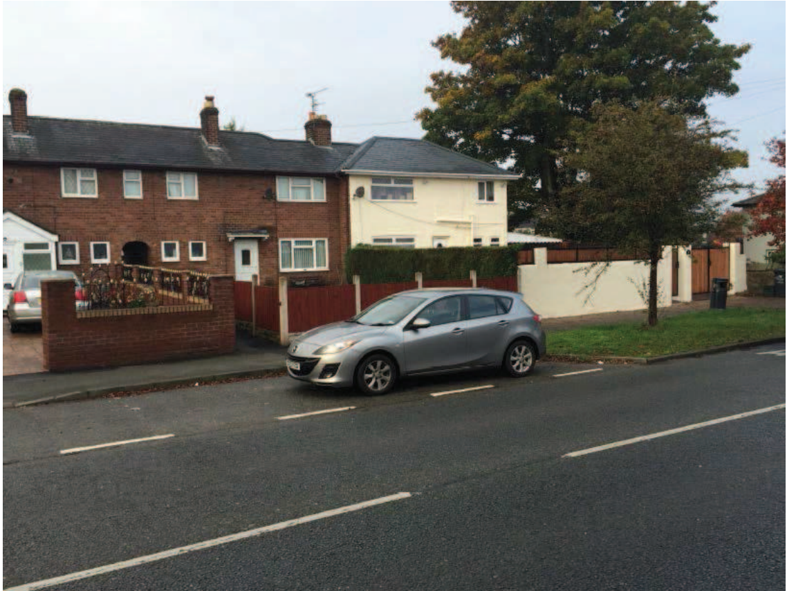
Application site frontage viewed from Stansty Road
