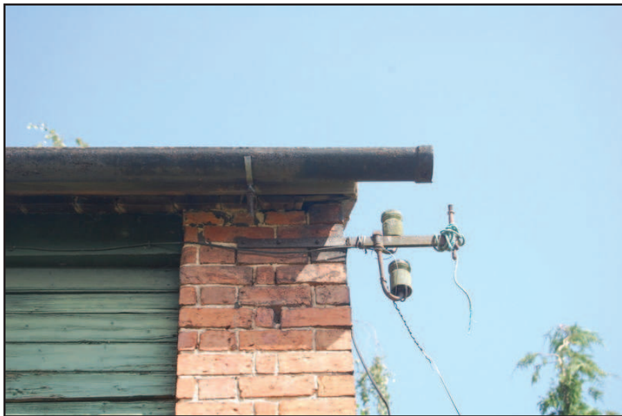
6. Gap in brickwork
